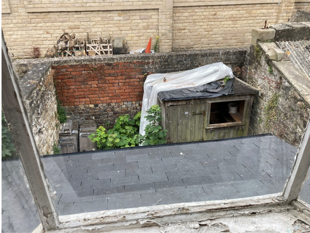
View of rear yard from bedroom window
