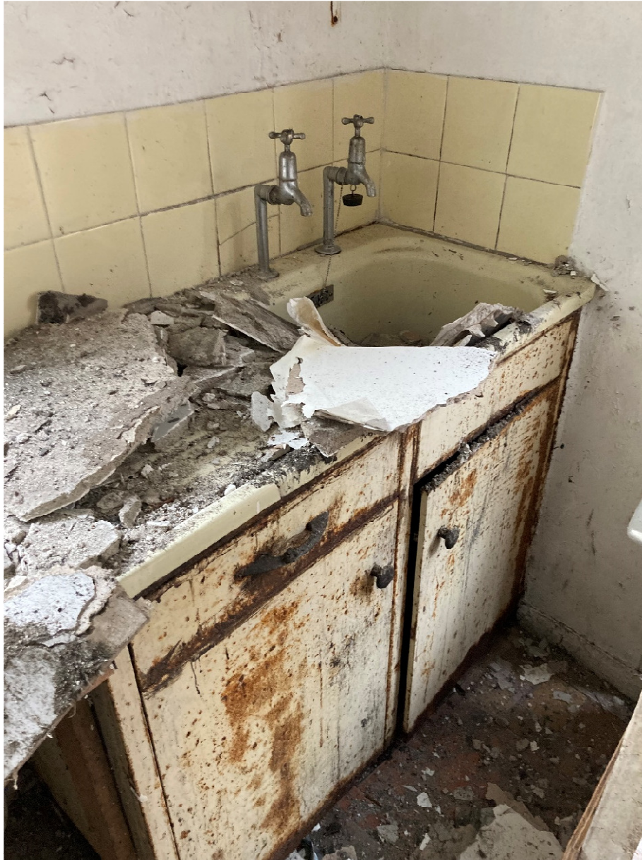
Image of existing metal kitchen unit
