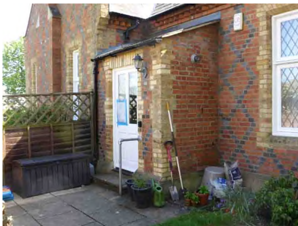
Figure 11: Early 20 th century lean-to on the northern side of the building (2018)
