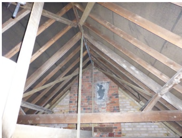
Figure 16: View of the roof structure over G7 (2018)
