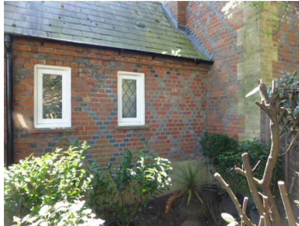
Figure 13: Infilled door opening on the north elevation at G10 (2018)
