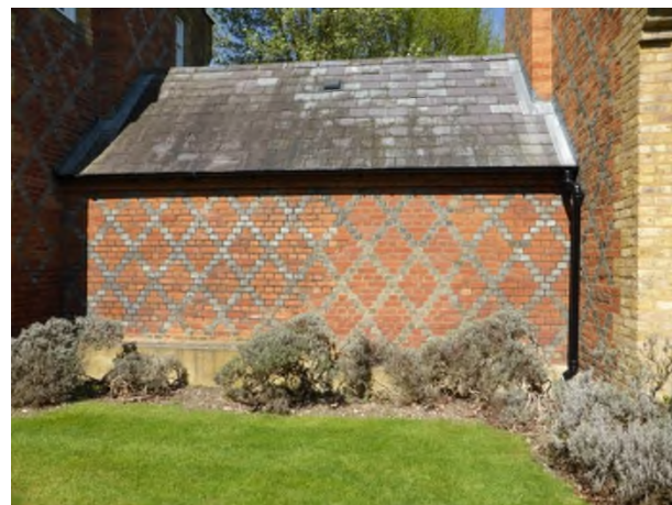
Figure 14: South elevation of the former Closets showing an infilled door opening (2018)
