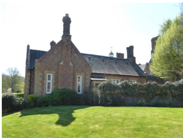
Figure 10: North elevation of 19 Bears Rails Park (2018)
