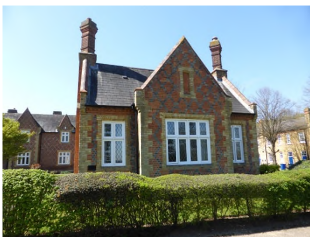
Figure 9: East elevation of 19 Bears Rails Park (2018)
