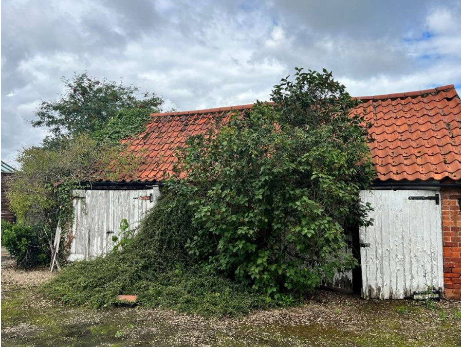
Photo 01 – Front Elevation (south)
