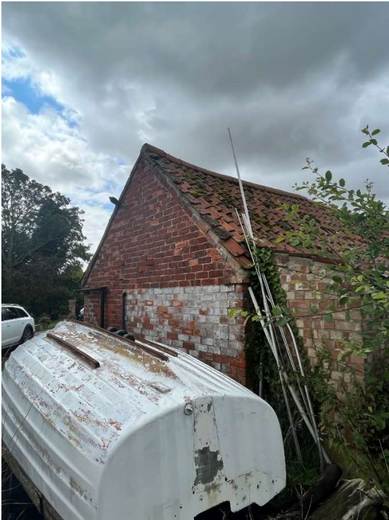
Photo 04 – Side Elevation (east)
