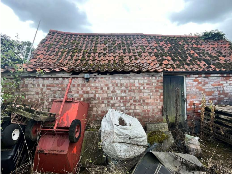
Photo 03 – Rear Elevation (north)
