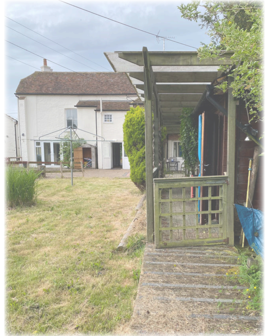
IMAGE 14 | Photo of Days Rooms Long View Towards Rear of Berkeley House
