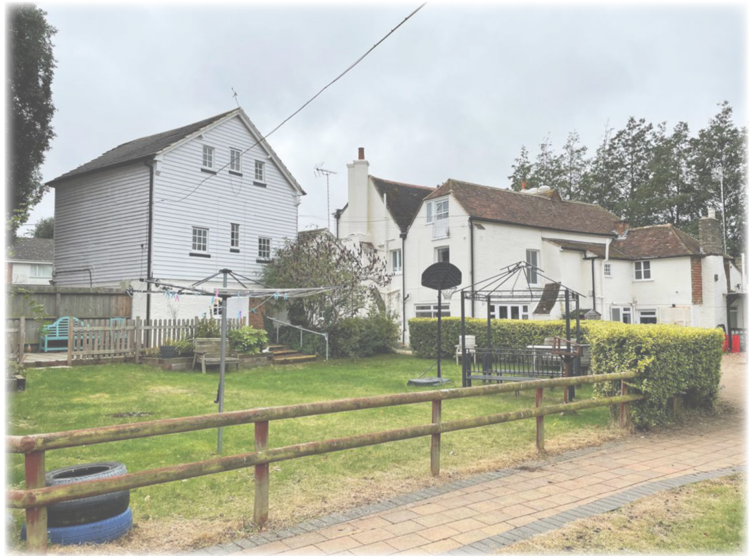
Photograph Towards Rear of The Mill (Left) and Berkeley House (Right)
