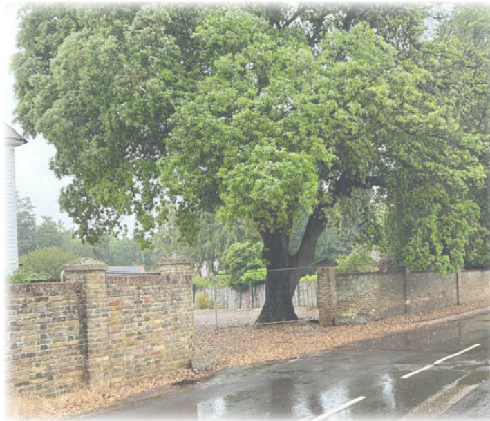
IMAGE 2 | Photograph of Front Boundary Wall | Existing Site Access
