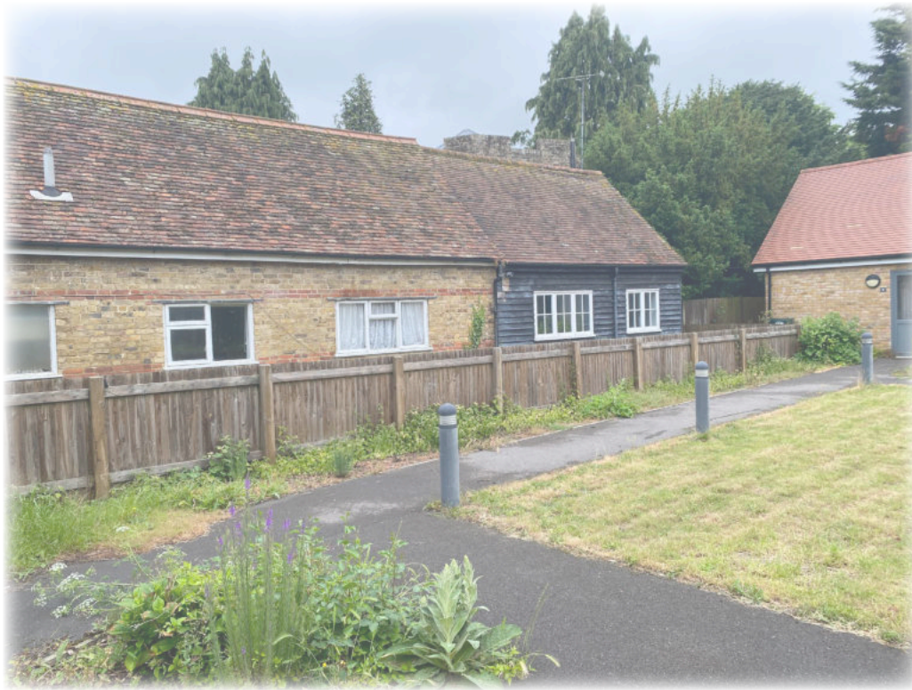
IMAGE 10 | Photo of Rear of The Windmill / Boundary Fence to Pippin House
