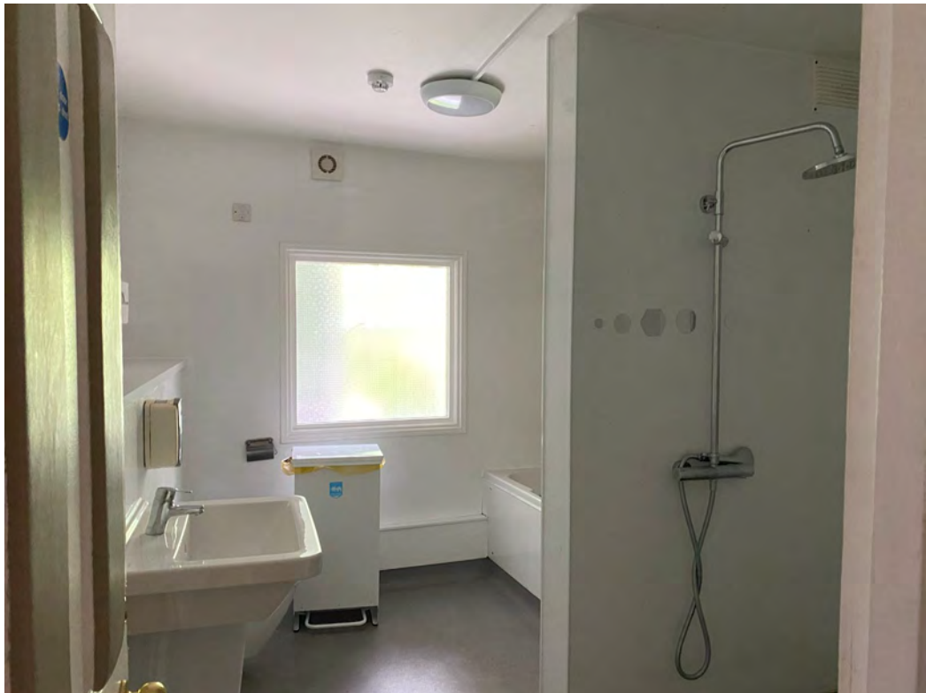
2.7: First floor modern bathroom with no external windows to be removed
