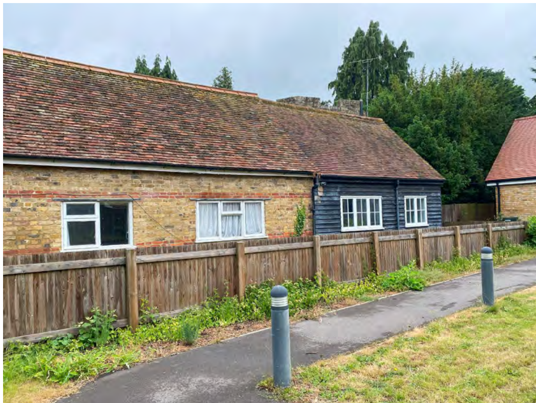
Fig. 28: Rear (east) elevation of early 20 th century additions to the smock mill base, which is just visible behind the weatherboarded addition. Pippin Cottage are to the right
