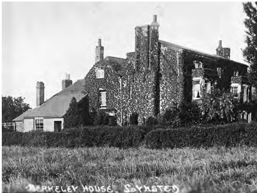
Fig. 14: Undated Photograph, Berkeley House from the south-west showing ivy covered west elevation and rear outshoot which looks to have been rendered and possibly reroofed.
