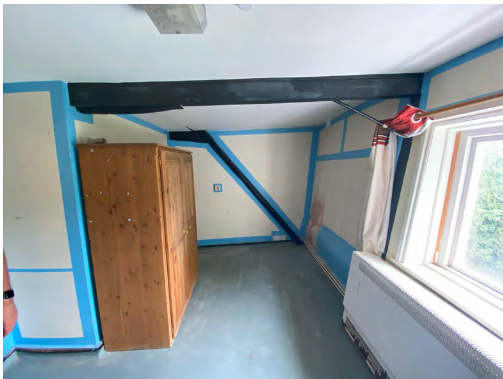
2.10: Second floor room with timber framing
