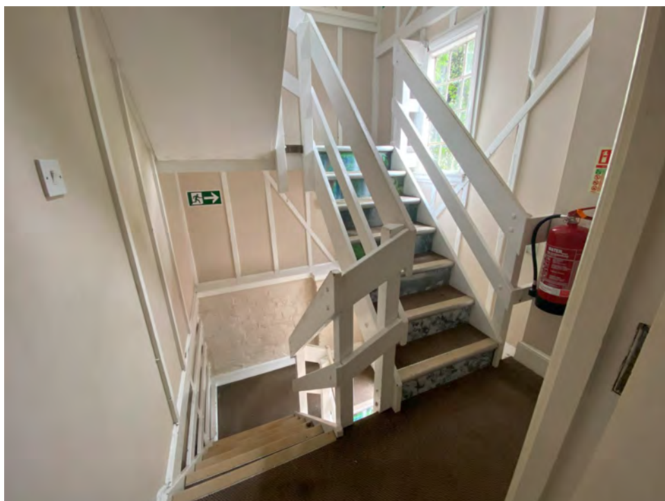
2.13: Modern staircase within mill serving all floors aside from basement
