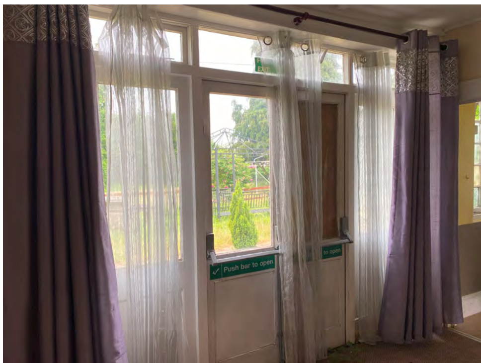
2.16: Modern fire doors to be replaced with timber framed French doors
