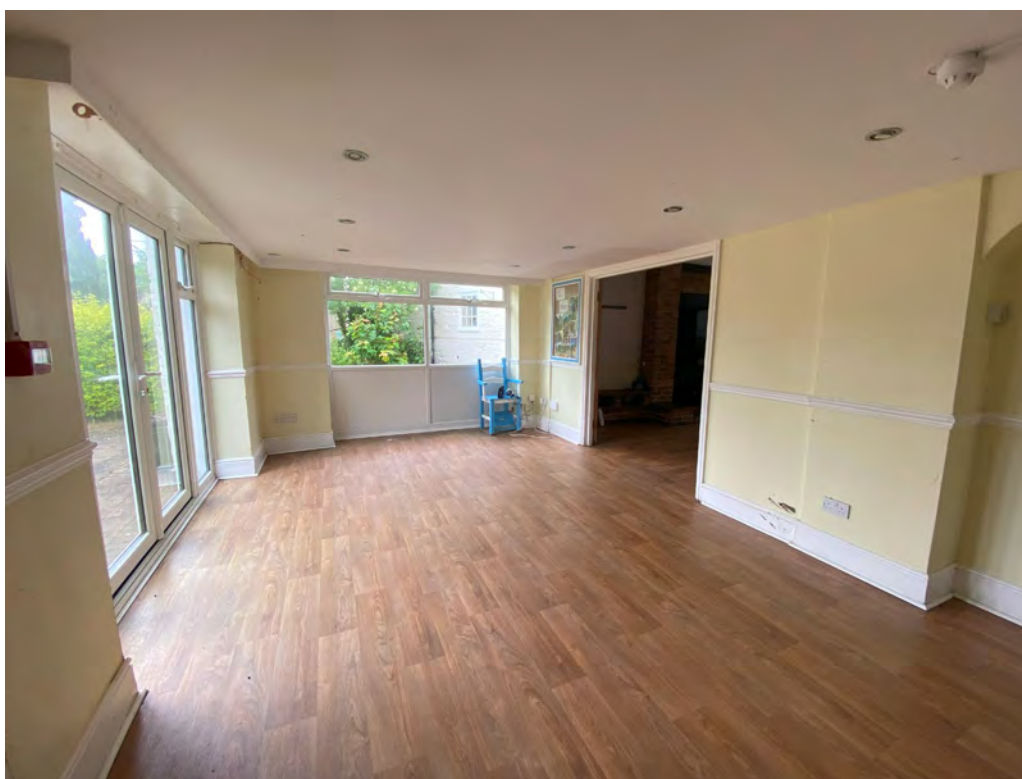
2.4: Plastic windows and doors to be replaced with better timber examples
