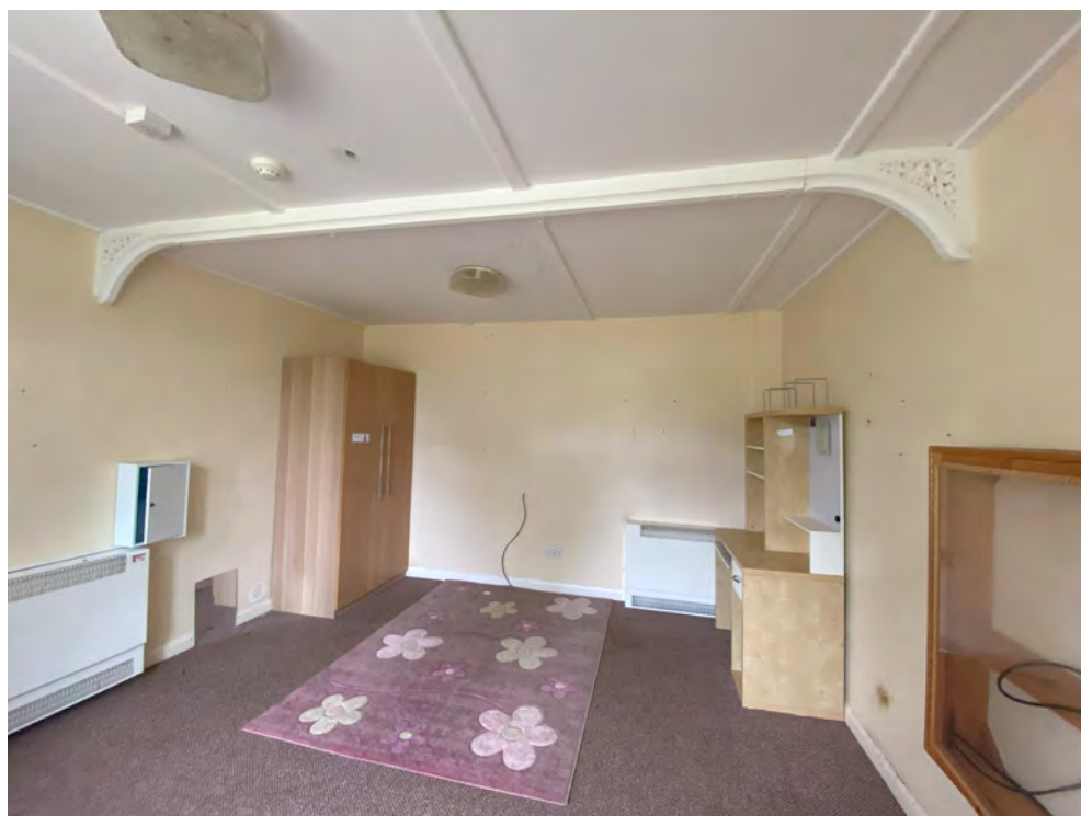
2.15: Ground Floor southern room with only decorative beam to be retained with new door to ensuite
