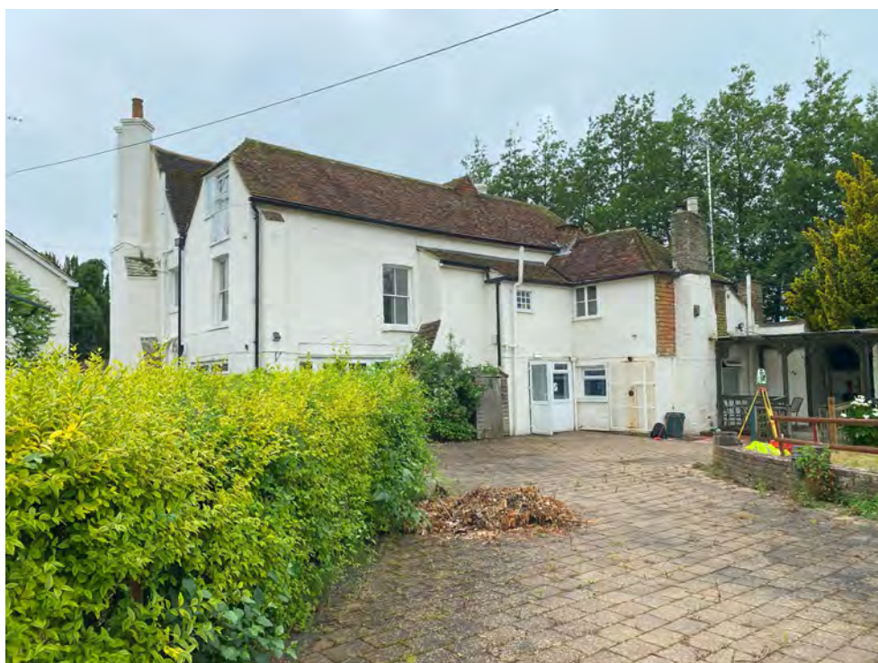
Fig. 22: Rear elevation of Berkeley House
