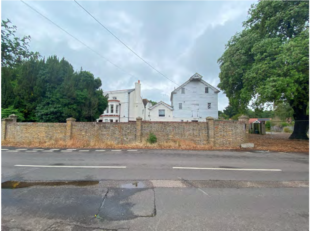
Fig. 25: View of both listed building directly south on Lynsted Lane
