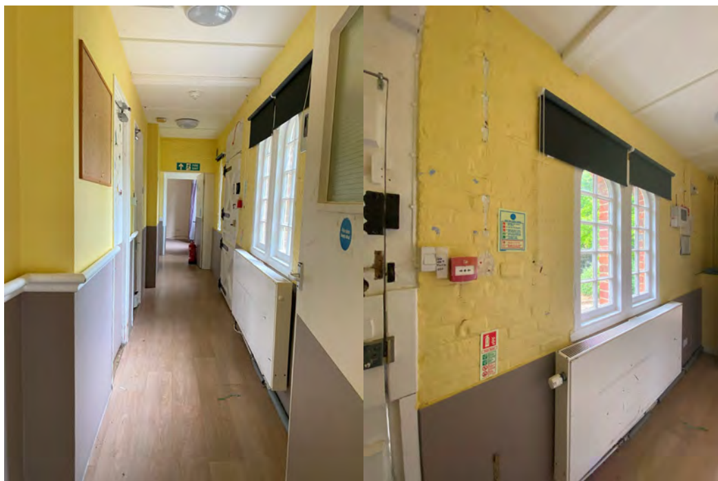
2.17: Existing corridor to be retained
