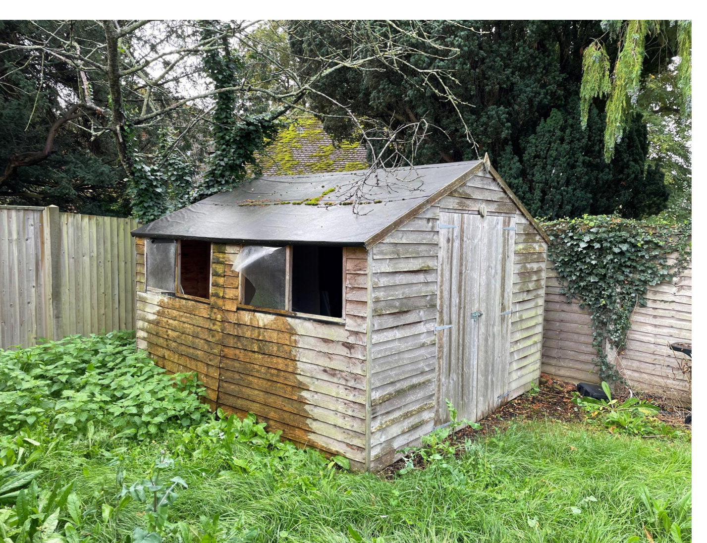
Outbuilding - E Timber Shed
