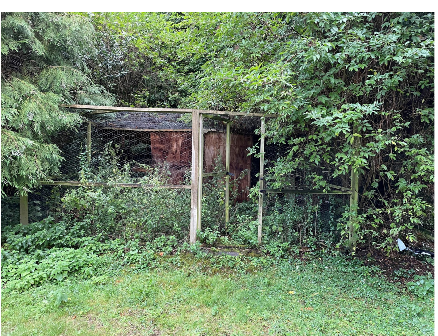
Outbuilding - C Chicken Coup - Meshed Timber Enclosure
