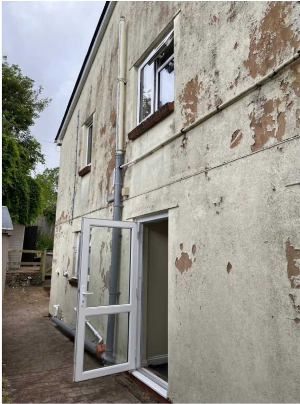
South Elevation and access into the corridor which accesses the staircase.
