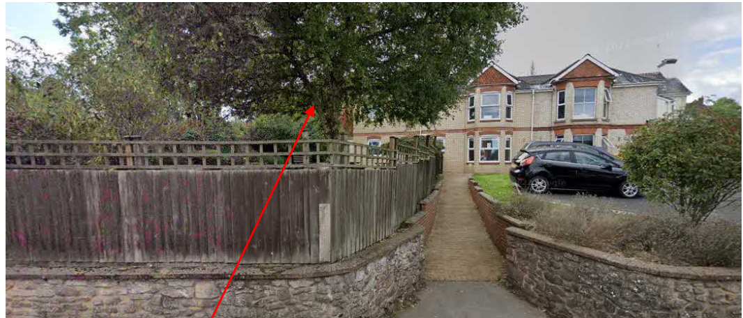
Site of proposed extension (not viewable from this view)
