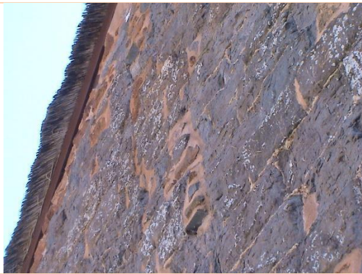
7. Crevices suitable for roosting bats at verge
