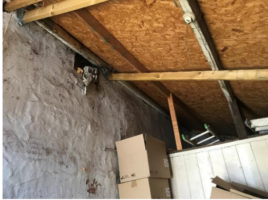
5. Ceiling void above boards (inaccessible) in extension
