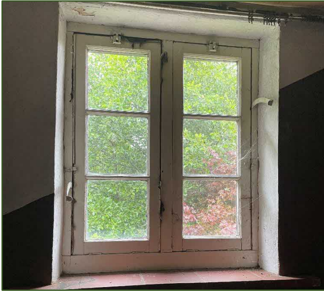
Figure 35. Workshop/store window (number 14) interior
