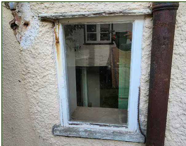
Figure 9. Kitchen window exterior
