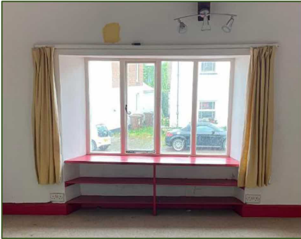
Figure 10. Bedroom 1 window interior
