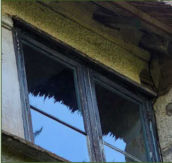
Figure 39. Landing window exterior
