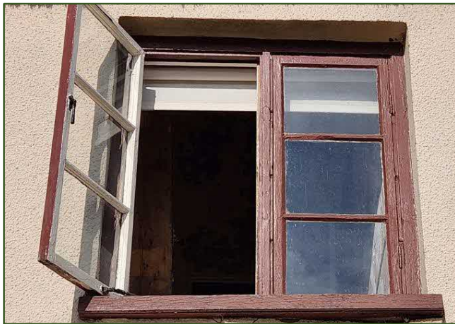
Figure 19. Family bathroom window exterior
