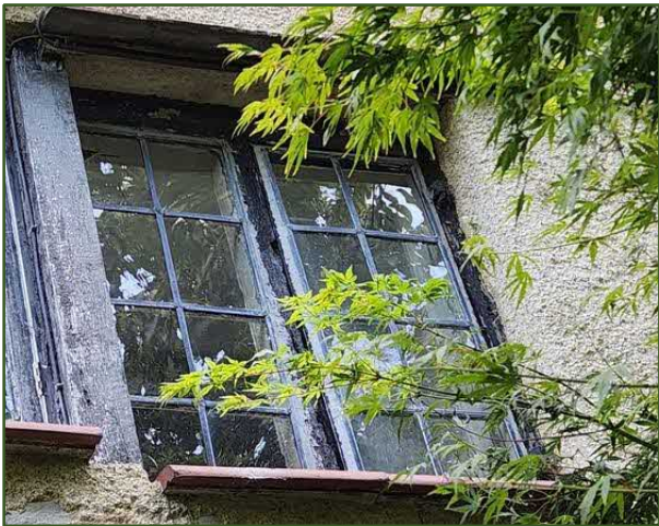
Figure 25. Under stairs space window exterior
