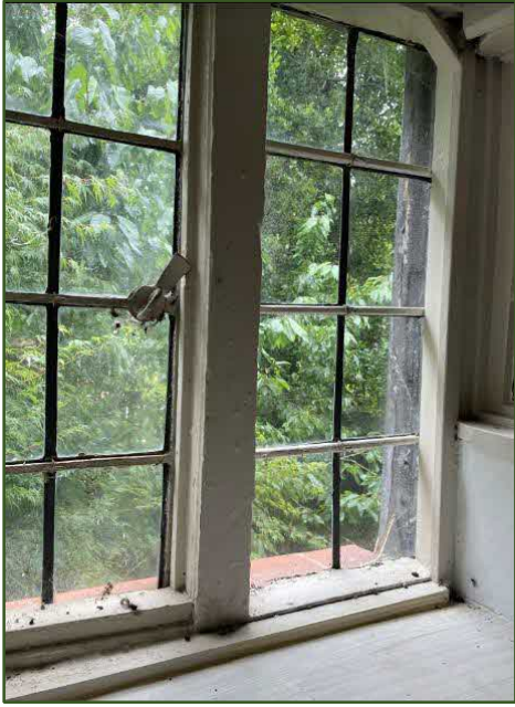
Figure 24. Under stairs space window interior
