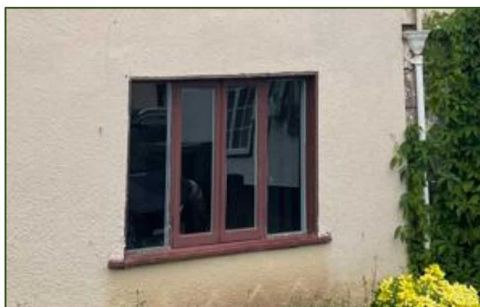
Figure 3. Sitting room window exterior
