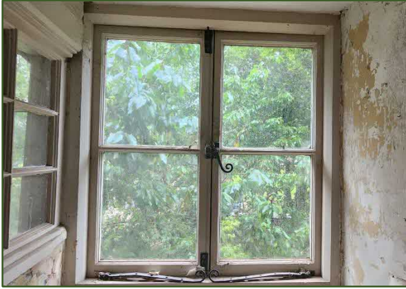
Figure 26. Dining room interior
