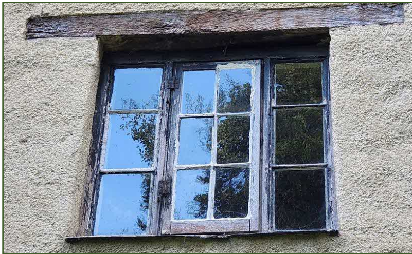
Figure 29. Kitchen window exterior
