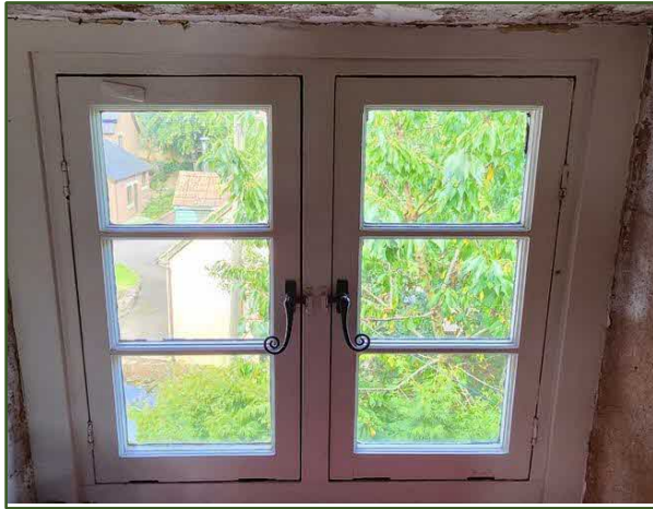
Figure 18. Family bathroom window interior
