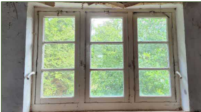
Figure 34. Workshop/store window (number 13) interior
