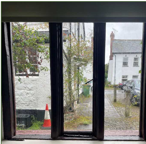
Figure 7. Dining room window interior
