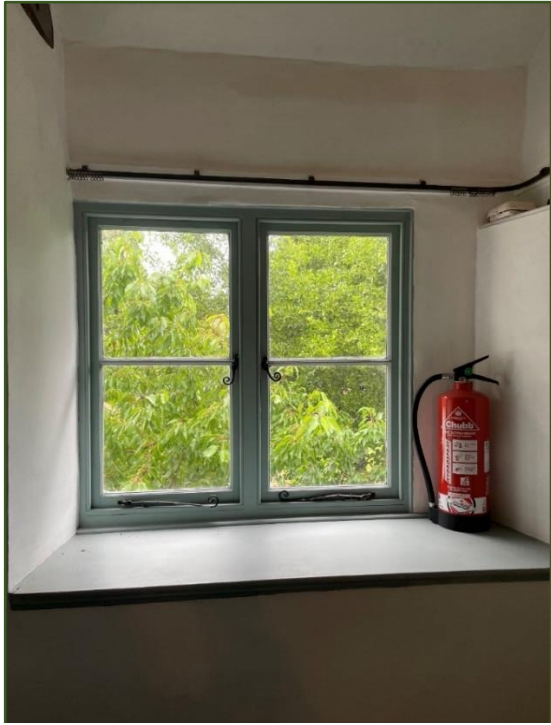
Figure 16. First floor landing window.
