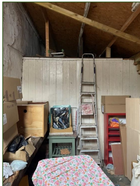
Figure 44. Interior of workshop/store looking towards timber infill.
