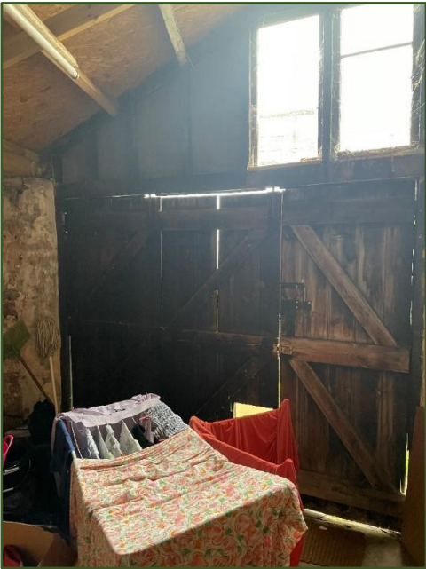
Figure 45. Interior of workshop looking towards front of building.
