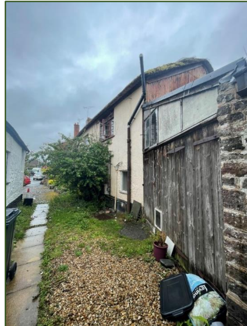
Figure 13. Southern elevation showing Workshop/store, southern gable end concealed with corrugated sheeting.
