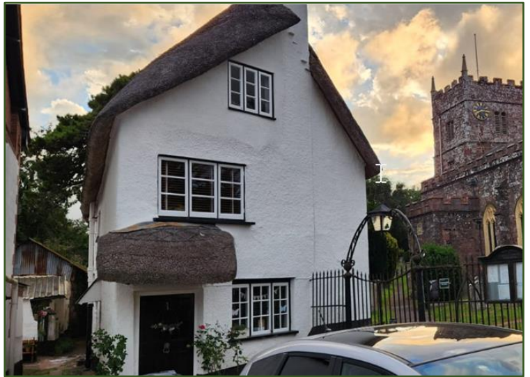
Figure 58. House within The Bury (opposite Abbotsford) demonstrating the style of window to be installed at Abbotsford.
