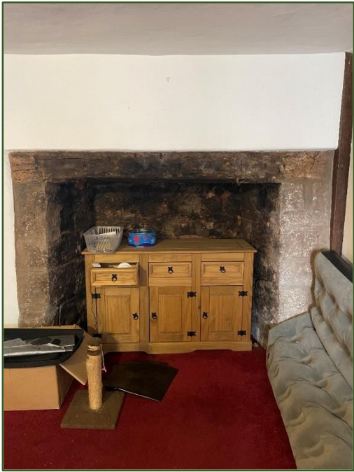
Figure 30. Dining room fireplace opening.
