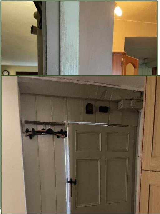
Figure 37. Kitchen doorway to corridor set within panel frame.
