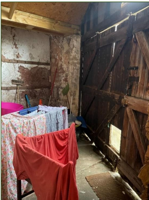
Figure 14. Workshop/store; timber doors.
