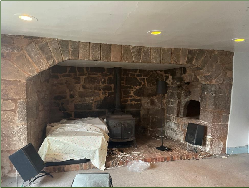
Figure 22. Fireplace (white asbestos register plate visible) with bread oven.
