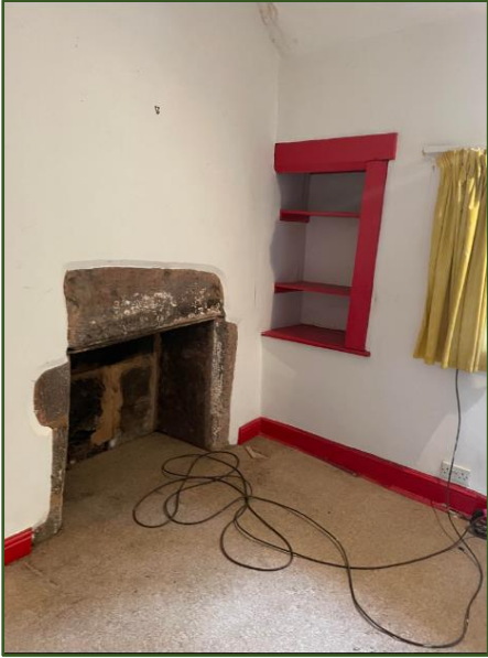
Figure 48. Bedroom 1 with stone fire surround and recess in wall.
