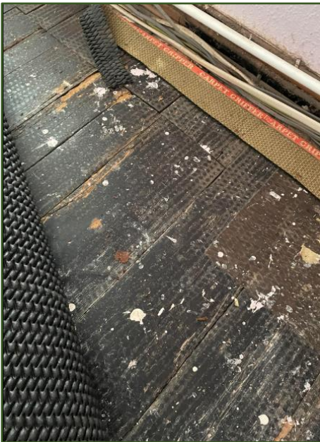
Figure 53. Elm floorboards first floor.
