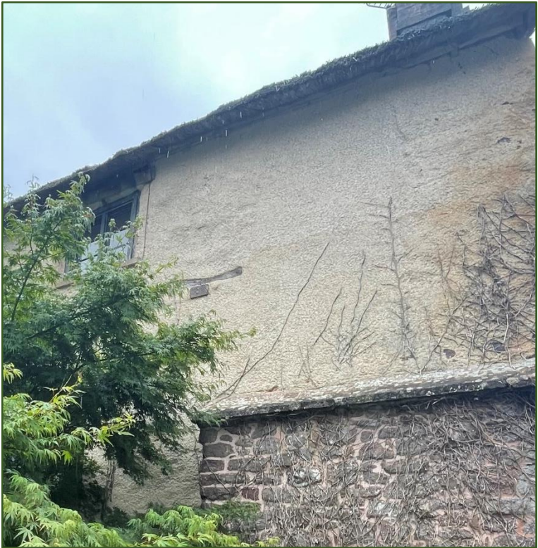
Figure 50. Indentations in render opposite bedroom 1 wall recess.
