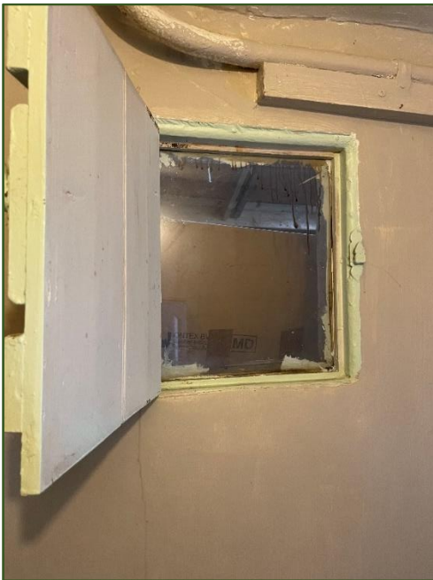
Figure 43. Historic window opening in original external wall (south) looking into workshop. Note wooden latch door.
