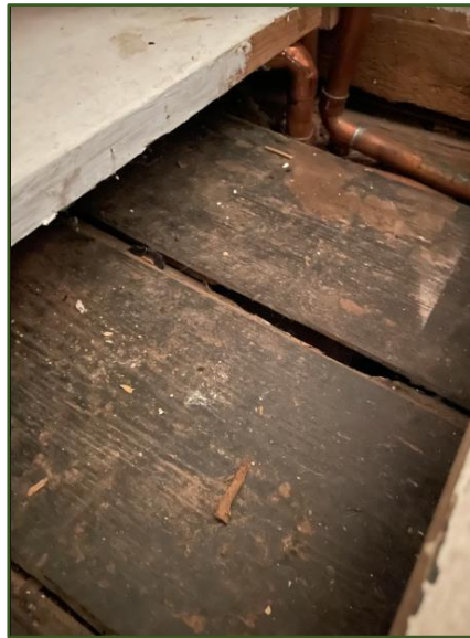
Figure 56. Elm floorboards set under later boards (first floor).
