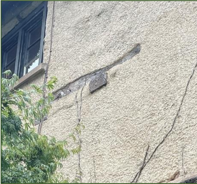
Figure 27. Rear wall with location of end of beam under lintel.
