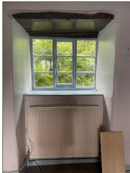
Figure 29. Sitting room window recess.
