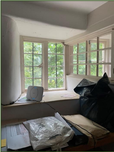
Figure 33. Understairs casement window with glazing bar and lead. Note internal window to right.
