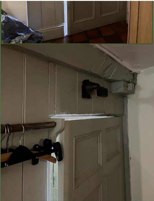
Figure 39. Kitchen doorway to corridor showing partial revealed southern beam.
