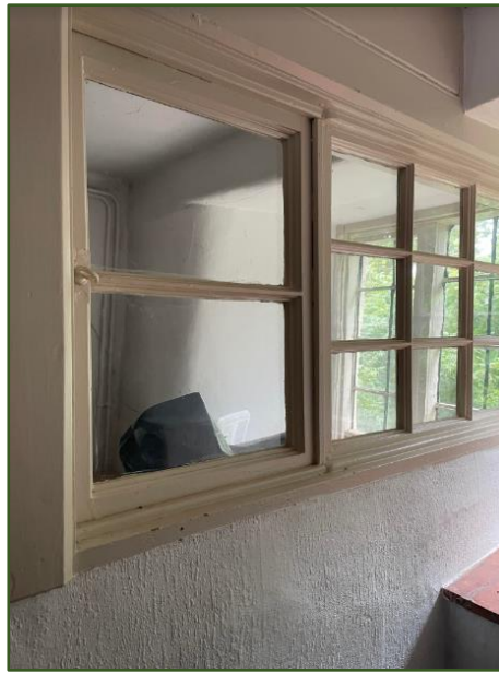
Figure 34. Internal window opening between downstairs and dining room.
