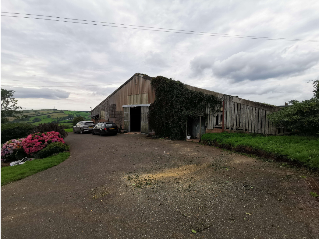
Existing barn building from South-East.
