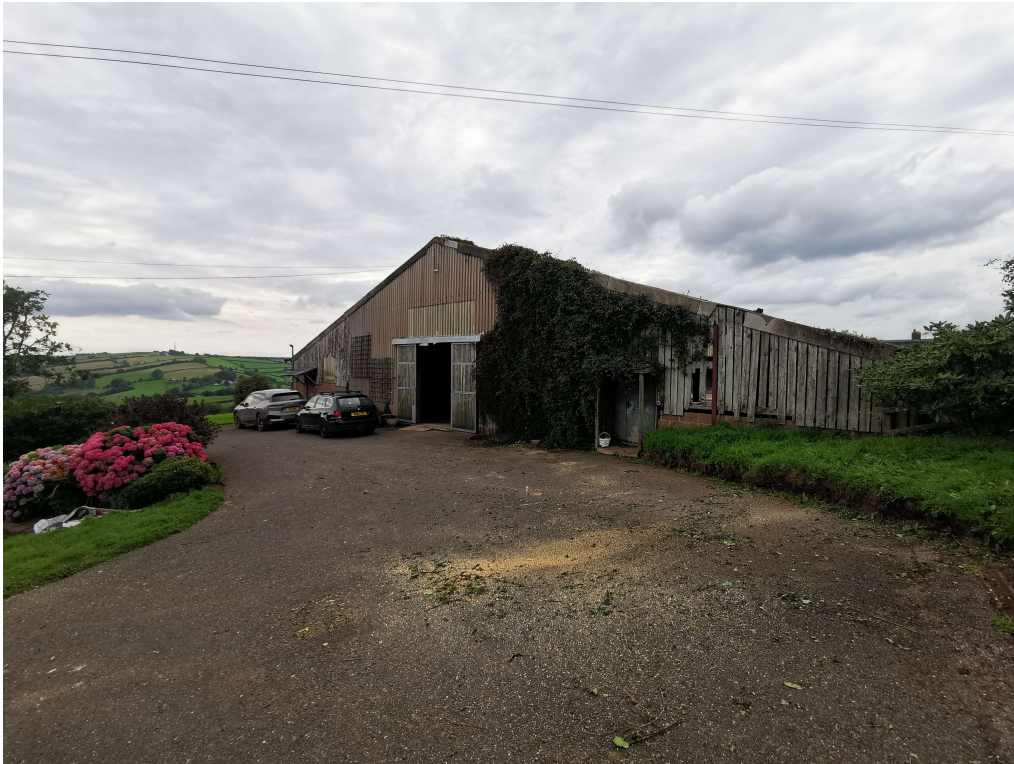
Existing barn building from South-East.
