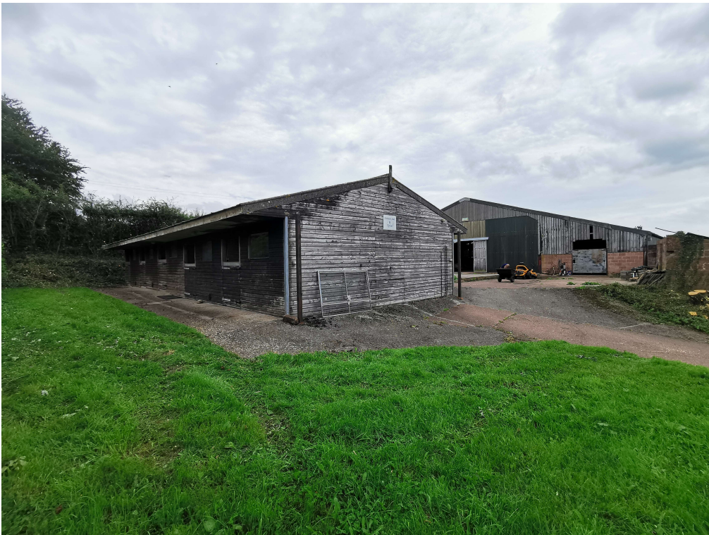
Existing stable and barn from North-West.
