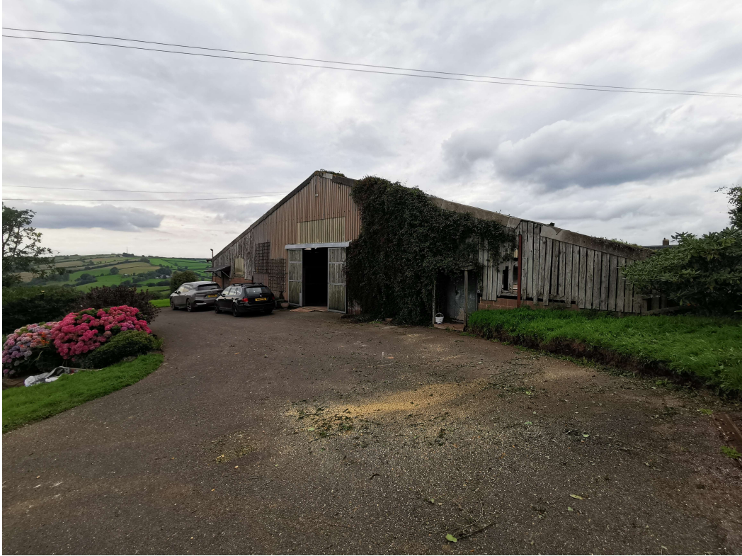
Existing barn building from South-East.
