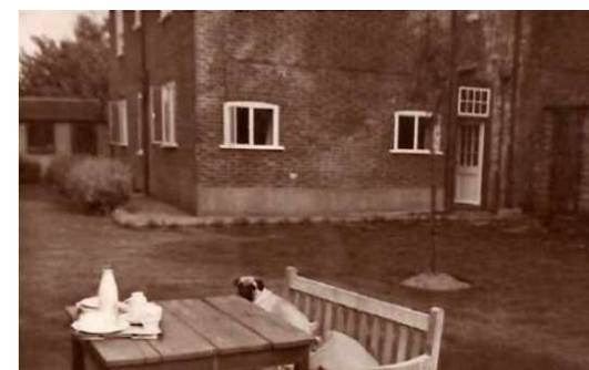
Figure 2. Photographs showing current west elevation and as was (including doorway proposed for reinstatement) in the 1960s
