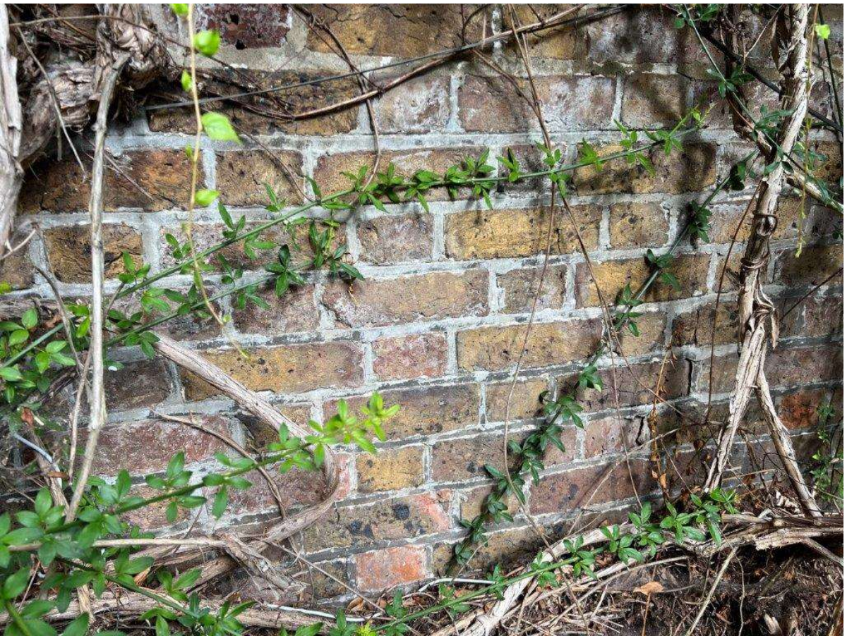
Photo of the existing garden wall
