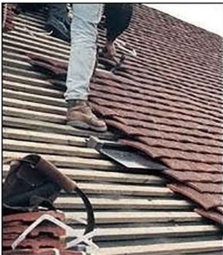
Concealed Vent outlet for mechanical extract units and SVP's
