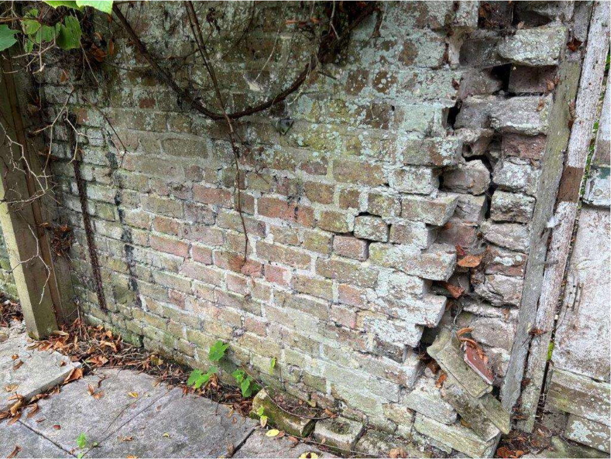
Photo of the existing garden wall
