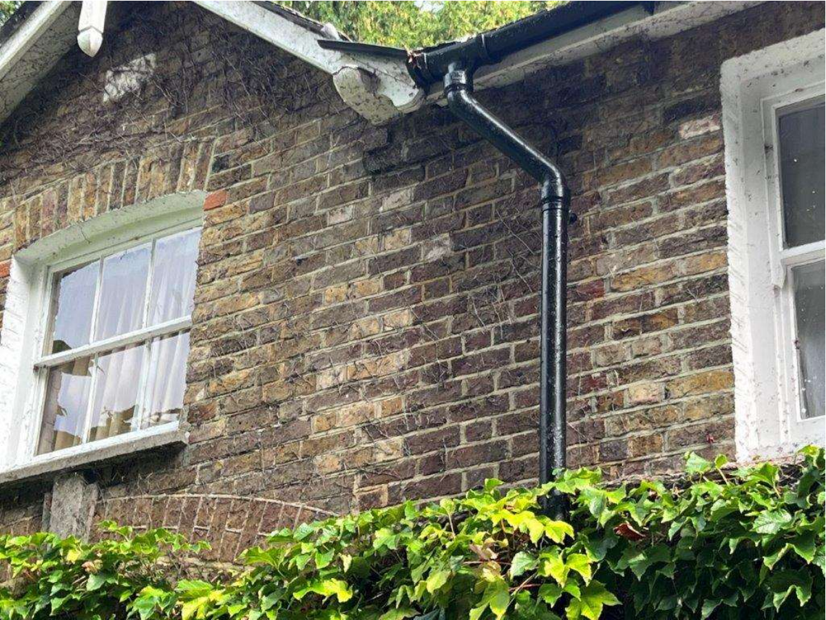
Photo of the existing Coach House
