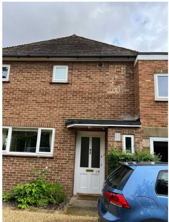
Figure 3. Site photo of existing entrance door.
