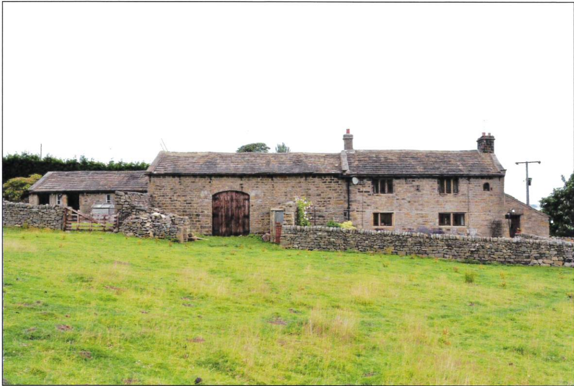
Photo 1: The farmhouse and barn range: south front
