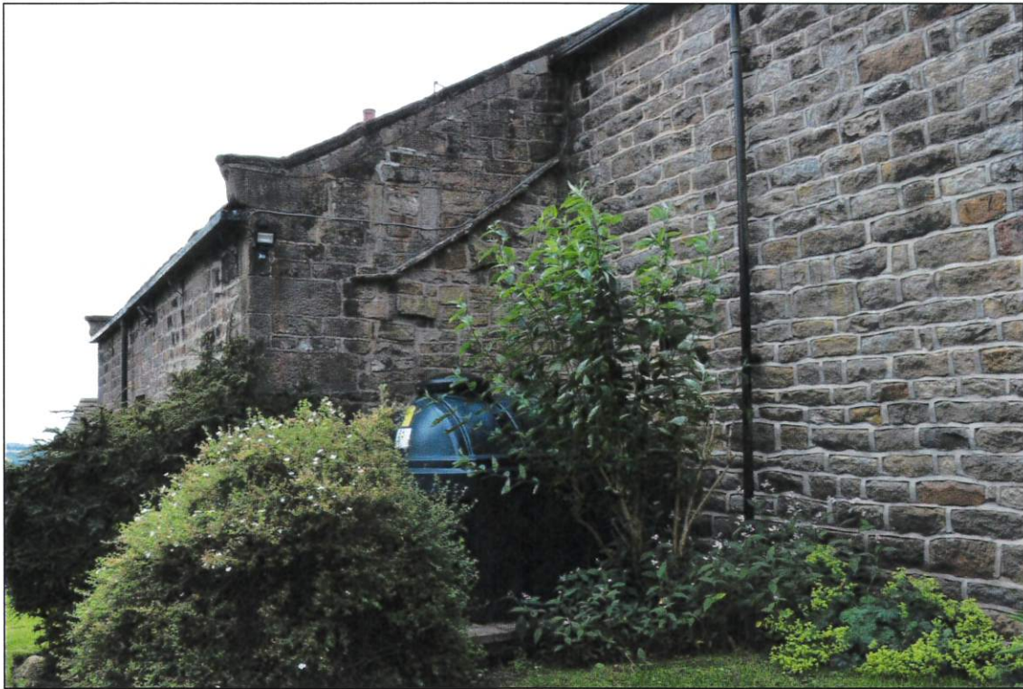
Photo 5: West end of outshut behind farmhouse; rear of barn to right
