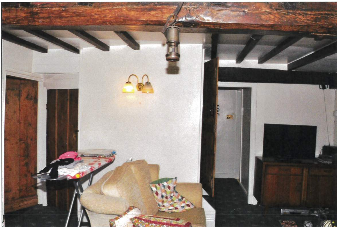
Photo 6: Living room/housebody, looking north; modern staircase projecting into room
