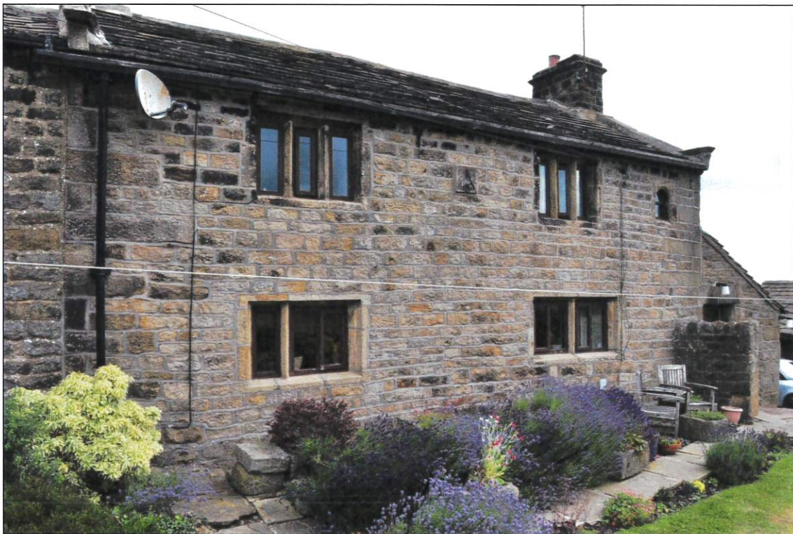
Photo 2: Farmhouse: south front
