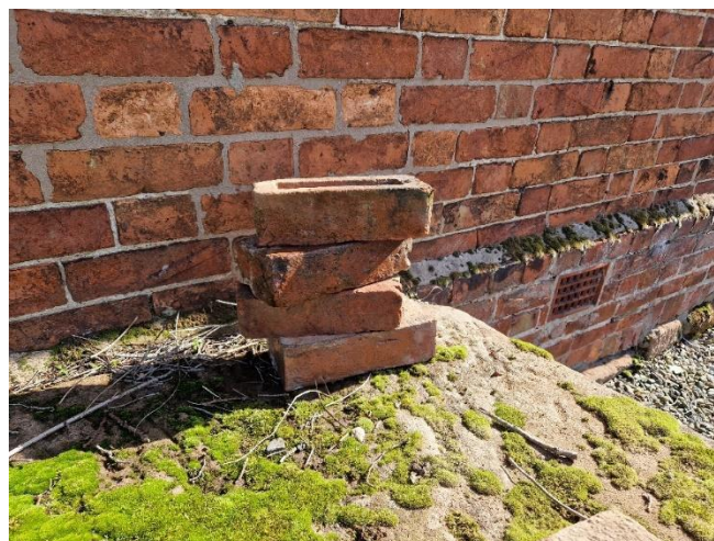
Image of the wall of Brades Farmhouse Bottom 4 bricks – reclaimed bricks from holding Top brick – Marshall Antique brick
