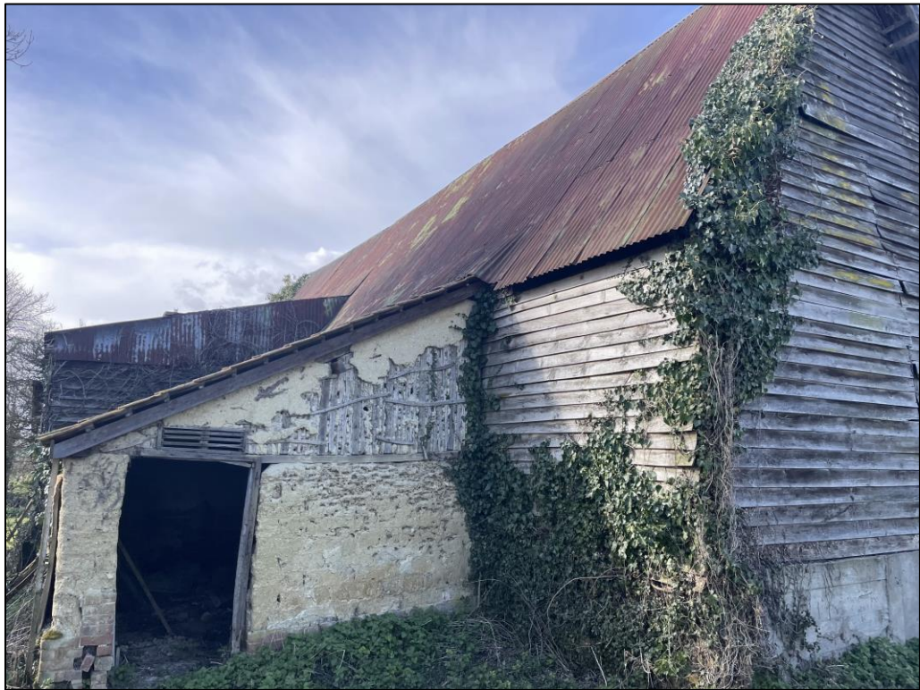
Figure 2.4 - Barn Viewed from the South East
