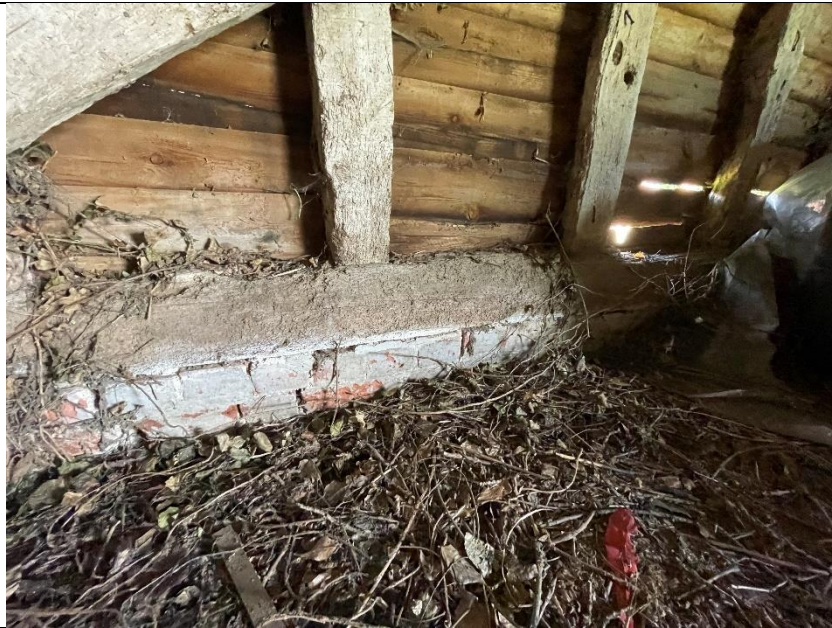
Photograph 11 Sole Plate West Elevation
