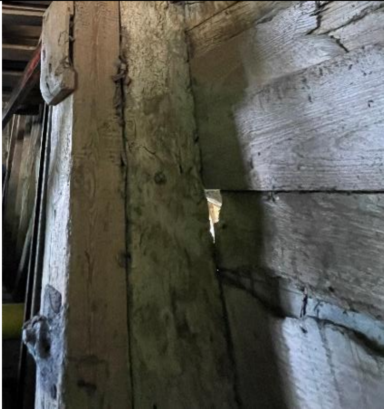
Photograph 15 Partner Repair to Post
