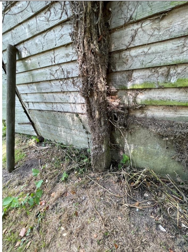
Photograph 08 Concrete Repair to Plinth South Elevation
