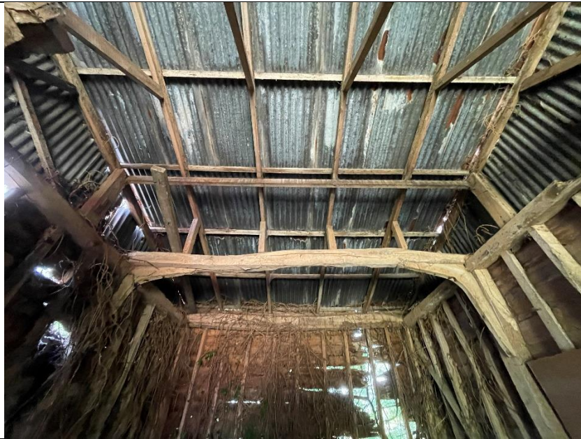
Photograph 19 Projecting Bay Roof
