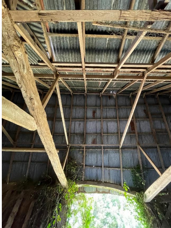
Photograph 17 Replacement Rafters Western Bays
