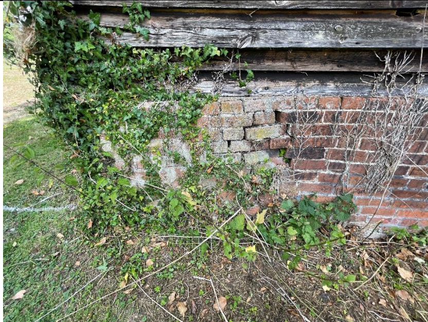
Photograph 06 Brick Plinth West Elevation
