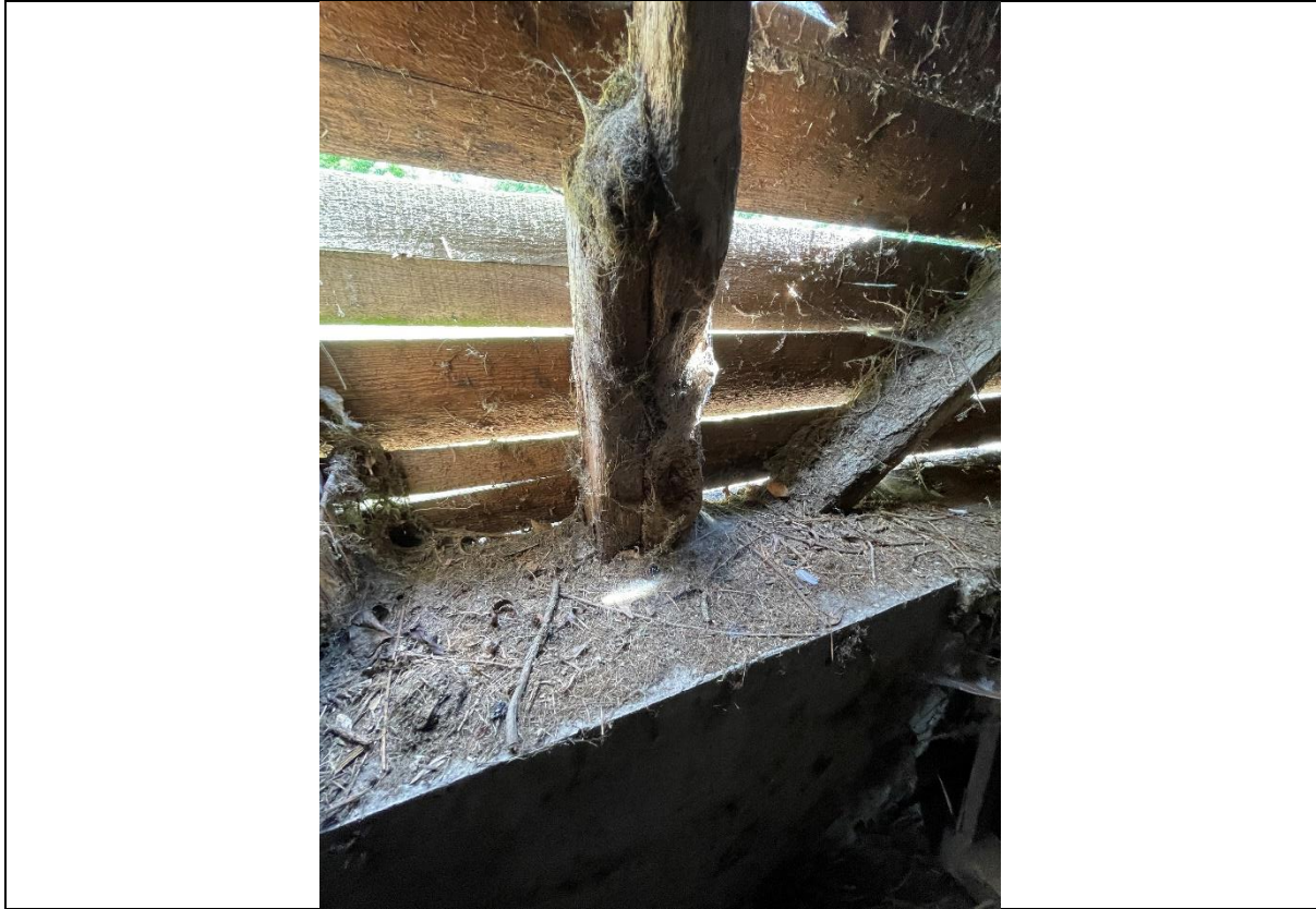
Photograph 13 Concrete Repair to Plinth and Partner Repair to Stud East Elevation
