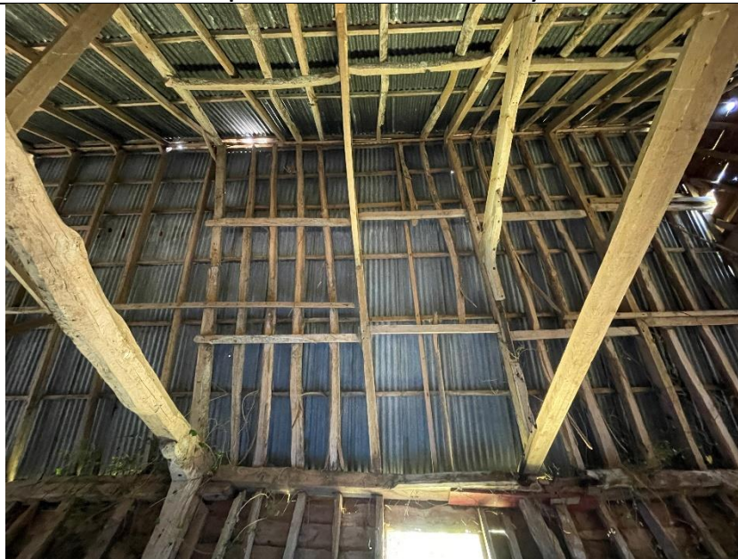
Photograph 18 Eastern Bays Racking to Roof
