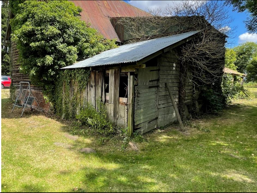
Photograph 23 Store South West Corner
