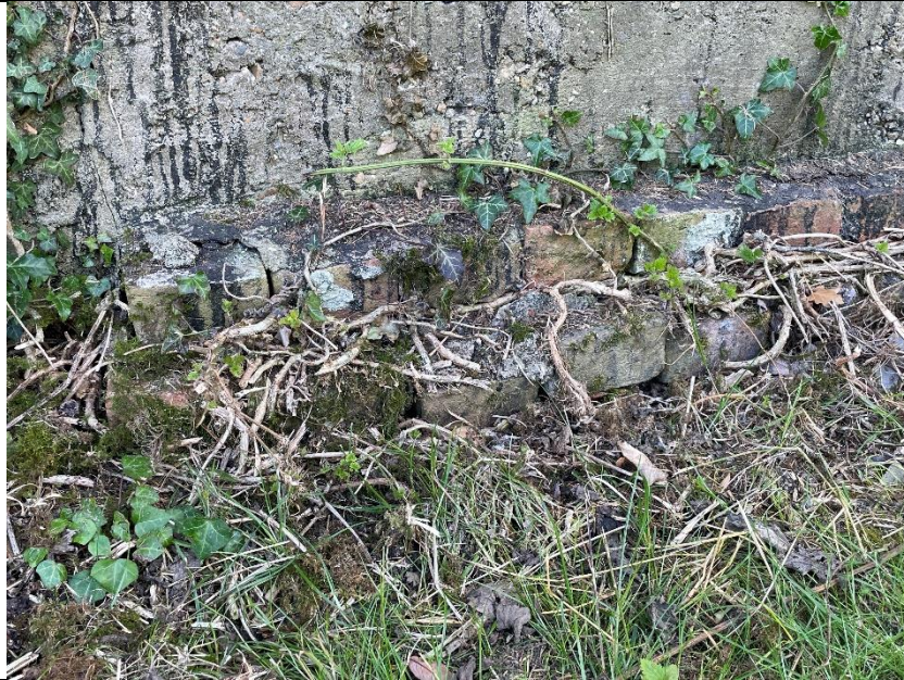
Photograph 05 Brick Plinth North Elevation
