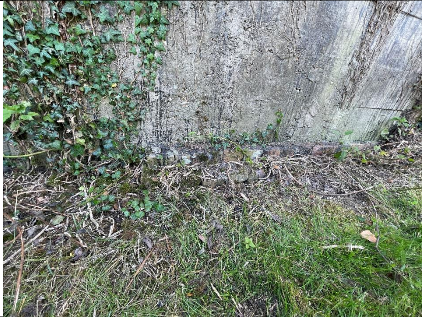
Photograph 07 Concrete Repair to Plinth North Elevation
