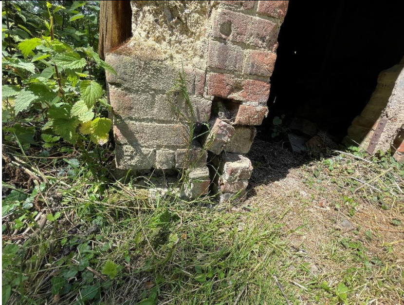
Photograph 10 Plinth South East Corner
