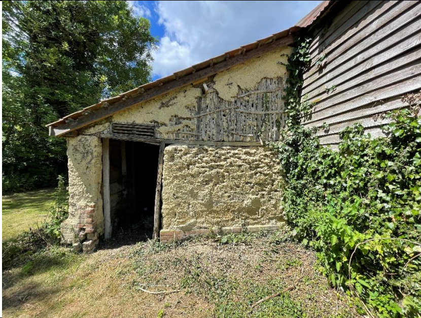
Photograph 09 East Elevation of Lean-To
