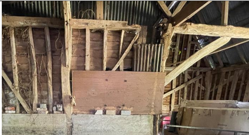
Photograph 20 West Wall of Projecting Bay
