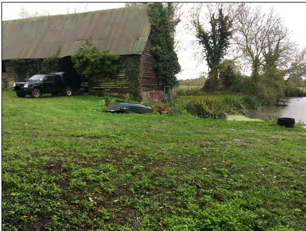
Photograph 4: The barn and pond immediately to the west of the site.
