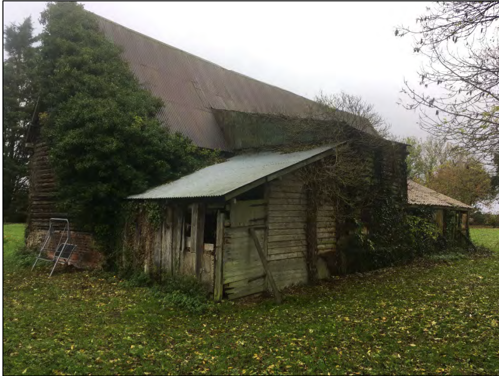
Photograph 15: The south-western side of the barn
