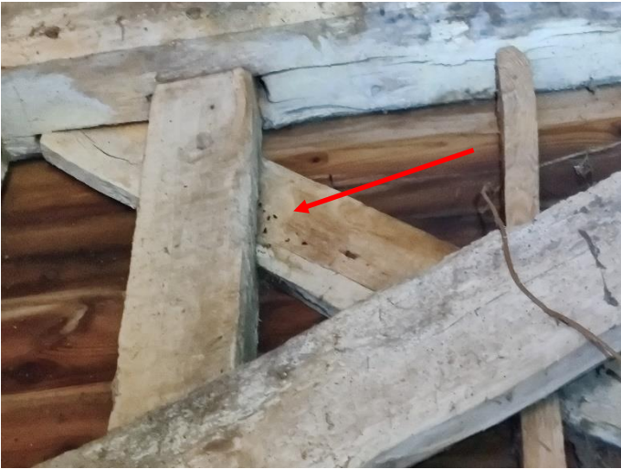
Photo 13 Bat droppings below open joint (roost) on internal wall (west)
