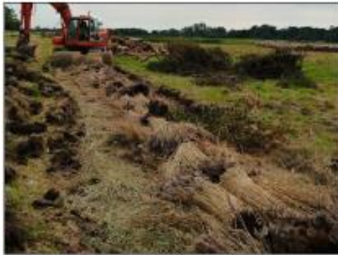
PHOTOGRAPH 1 - CENTRAL CORE PLACED OF REED BUNDLES AND RUSH BALES
