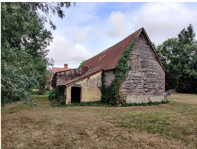
Photo 3 Southeast elevation of barn
