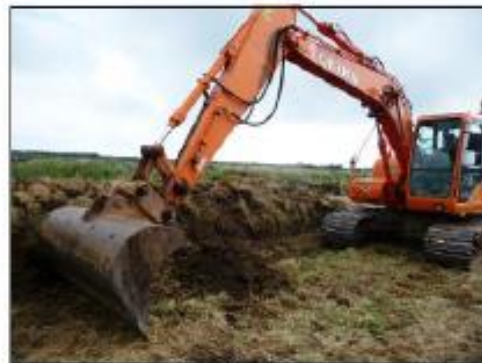
PHOTOGRAPH 4 - EXPOSING OF TIMBERS ON SOUTH FACE
