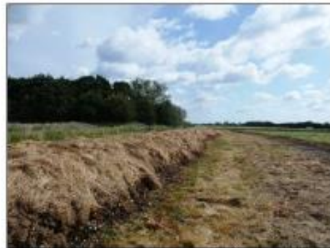
PHOTOGRAPH 6 - COMPLETED HIBERNACULUM BANK
