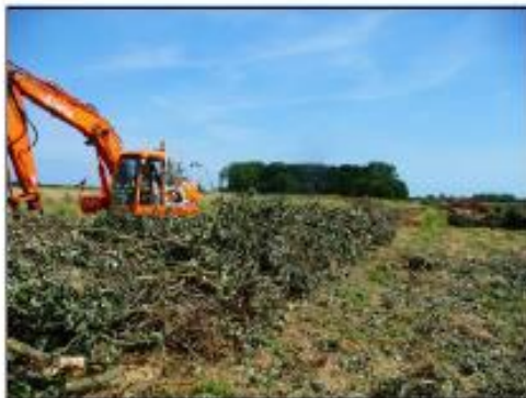
PHOTOGRAPH 3 - BRASH PLACED OVER REED BUNDLES AND LARGE TIMBERS
