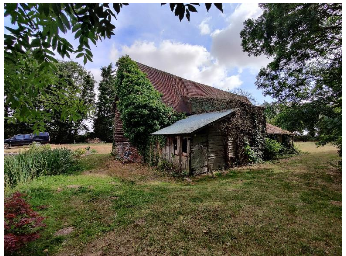
Photo 4 Southwest elevation of barn
