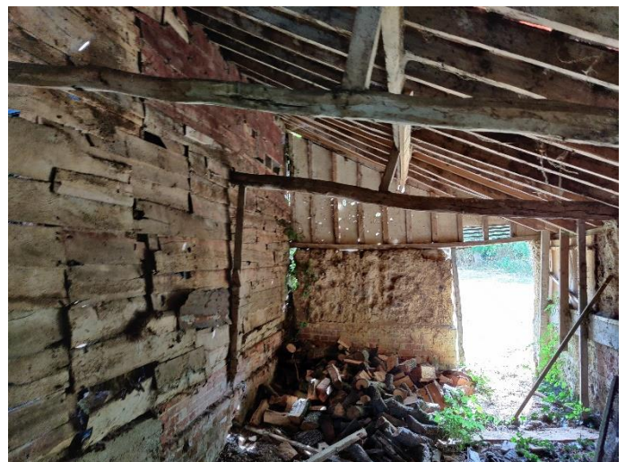
Photo 6 Internal view of attached store/lean-to section of barn
