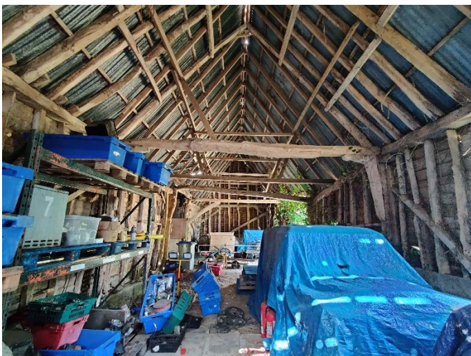
Photo 5 Internal view of main barn
