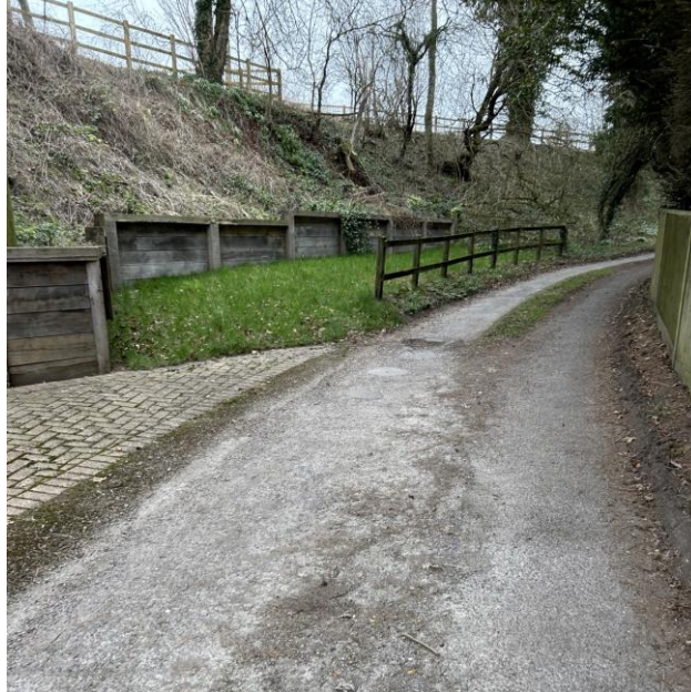
Photo 8: Example of existing access/parking on Mount Pleasant Lane
