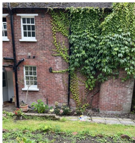
Photo 22: North side of the house (red brick), facing the wall
