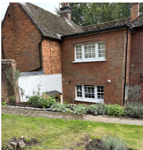
Photo 21: North side of the house (red brick), facing the wall
