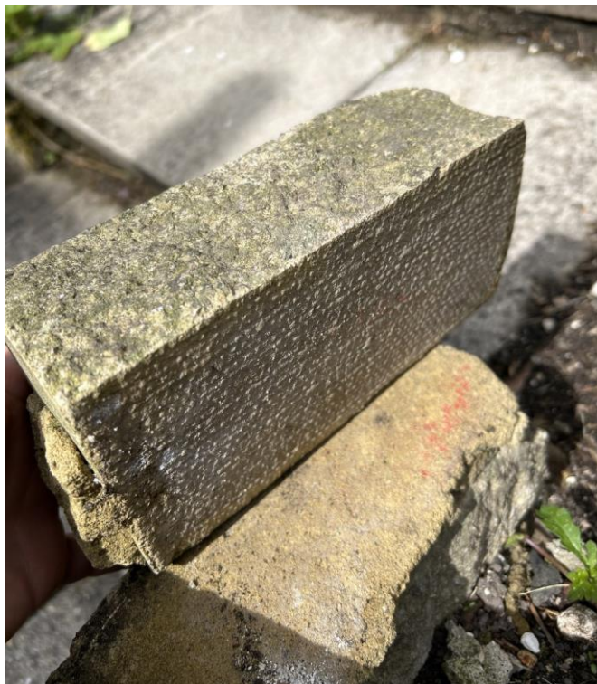
Photo 23: close-up of existing bricks
