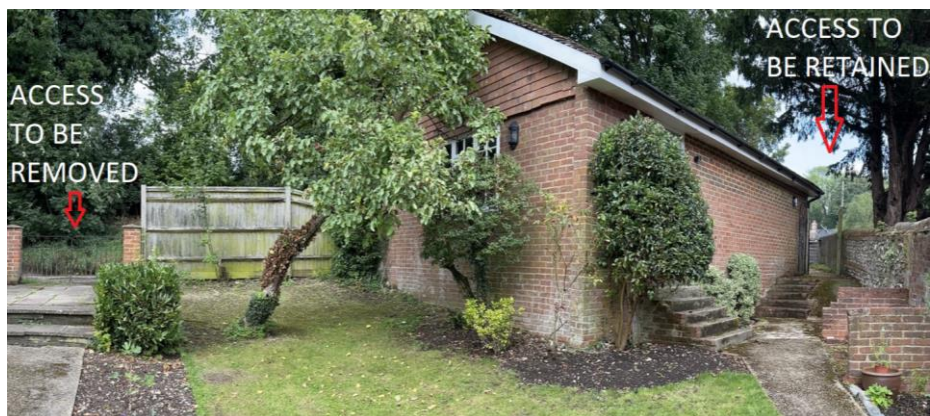
Photo 16: Two existing access points on Mount Pleasant Lane
