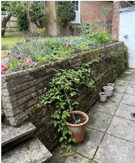
Photo 19: Exterior wall (looking north-east)
