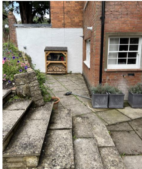
Photo 20: Exterior wall (looking east, showing the diagonal angle of the wall)
