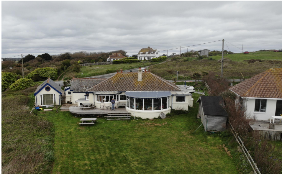
Existing Big Blue from the South side showing relationship with neighbour to the Eastern side.
