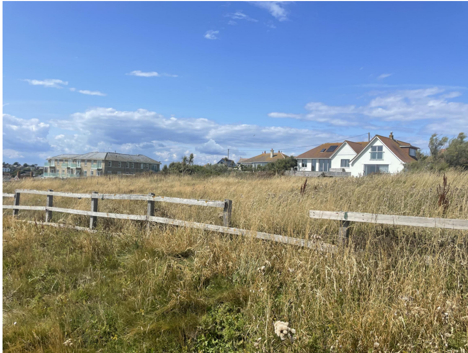
Marine Villa viewed from the South side showing prominent gables and glazing on this Elevation. Big Blue and St Martins Flats shown in the background.
