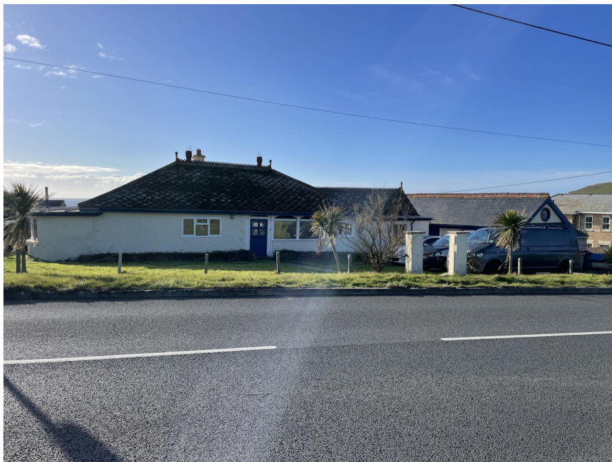
Existing Big Blue from the North side.
