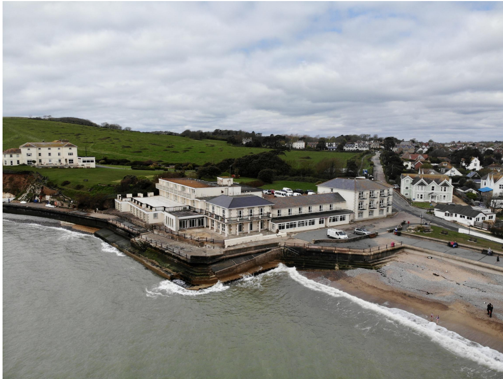
The Albion Hotel. Big Blues third neighbour on the South side. Again huge scale and mass, extensive glazing on all sides.
