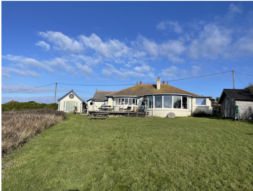
Existing Big Blue from the South side.
