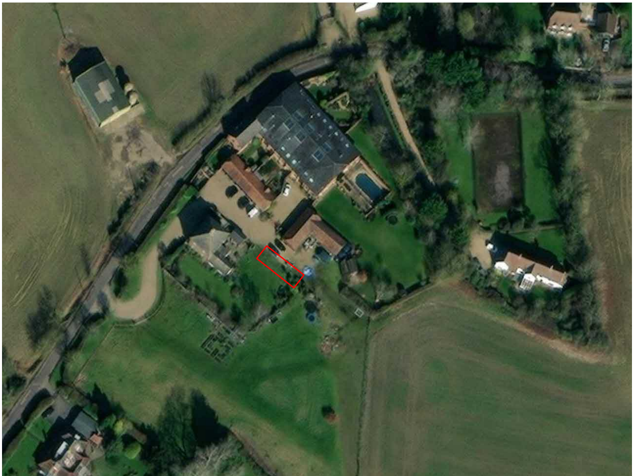
Aerial view of Uffords Farmhouse and Hunts Barn conversion and outbuildings
