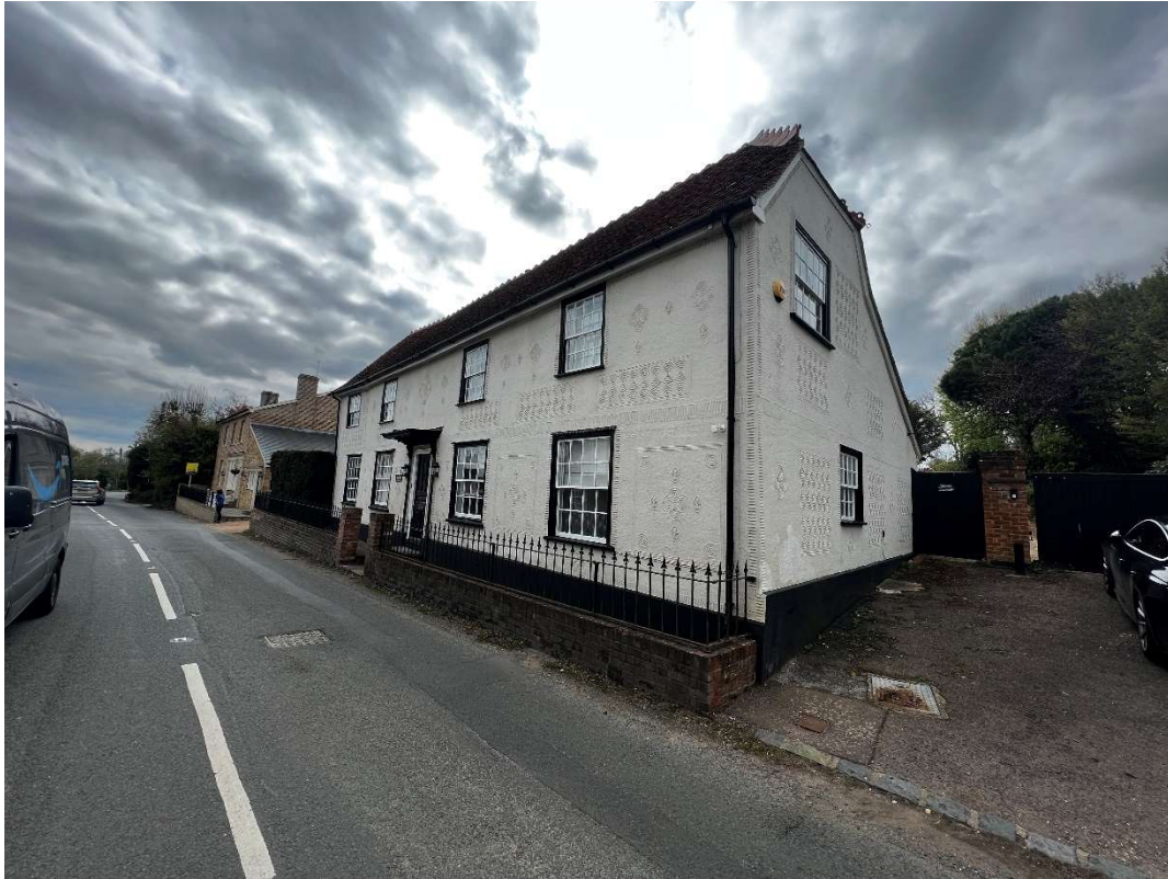
Front viewed from the north
