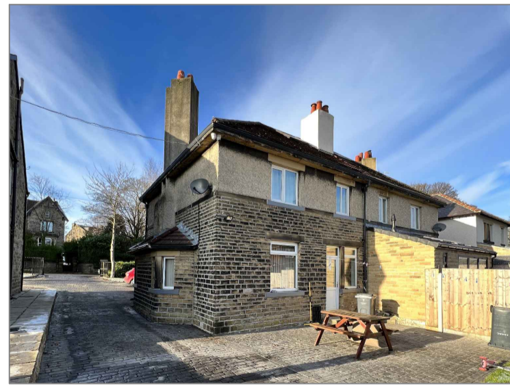
Photo 03 Showing Side & Rear Elevations
