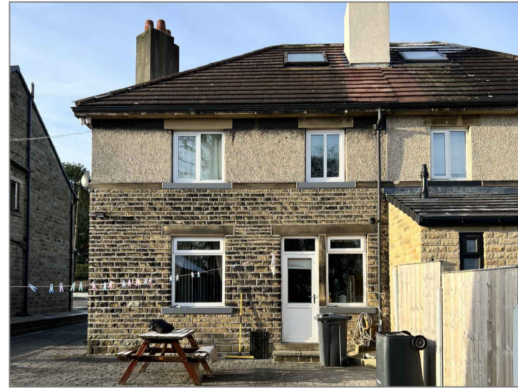
Photo 04 Showing Rear Elevation
