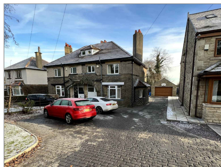
Photo 01 Showing Front Elevation
