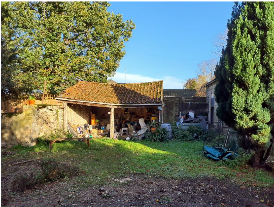
Figure 1 – Existing car port.
