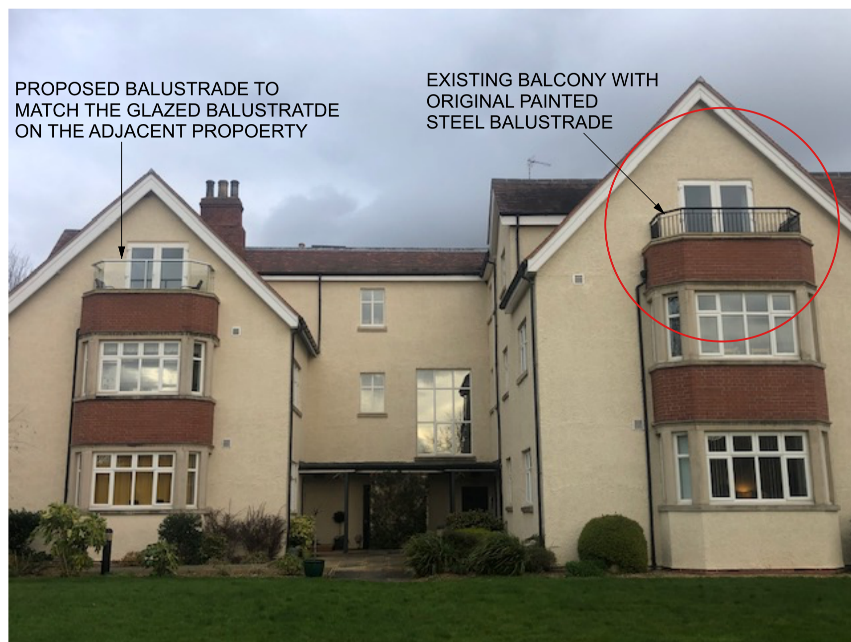
PHOTO OF WEST ELEVATION
