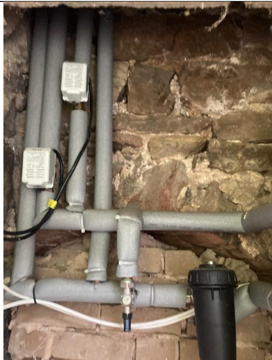
Plate 7 – internal stonework in boiler room
