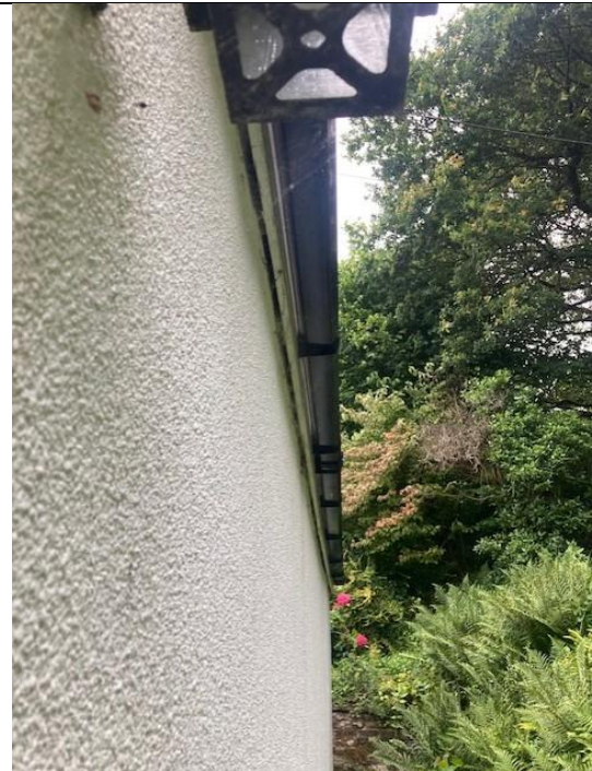
Plate 2 – facias on the northeast elevation of the garage
