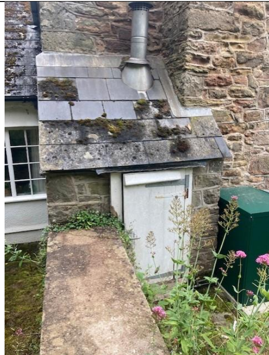
Plate 6 – external boiler room on northwest elevation
