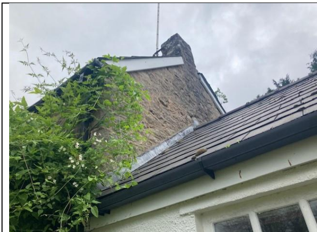
Plate 9 – Facias on southeast elevation of cottage
