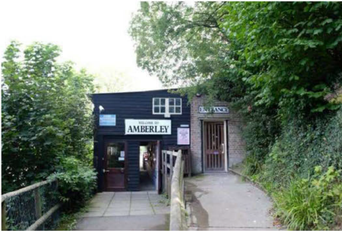
Photo 1. Bagging shed – public entrance, viewed from W.
