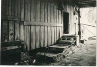
Photograph of the Bagging Shed taken in 1978 showing the opening to be reinstated
