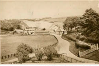
Photograph of the Bagging Shed taken from down the road by the station showing the open end of the shed
