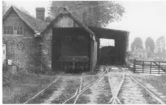
Photograph of the Bagging Shed looking from within, what is now Amberley Museum
