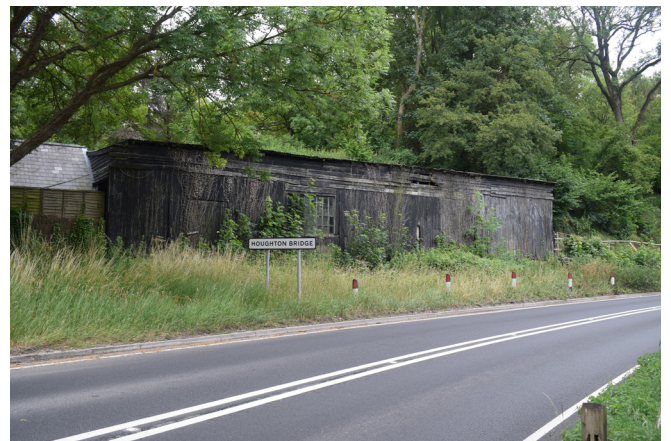
Fig 3. South elevation of loading bay
