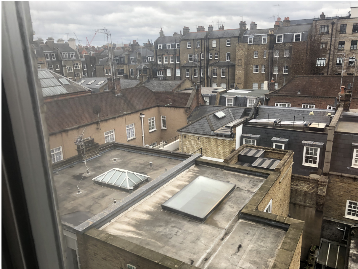
View from no 57 looking across no 55 to the rear.
