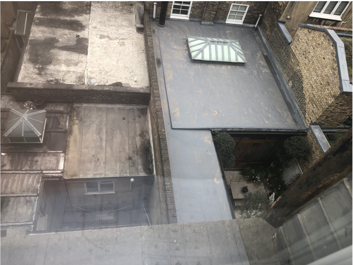
View from no 57 looking across no 59 to the rear.
