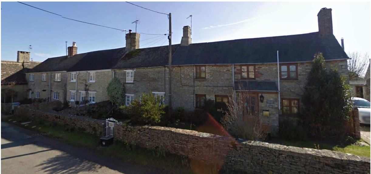
Fig 4. Terraced cottages being nos.101-106 Lower End immediately to the West of the application site
