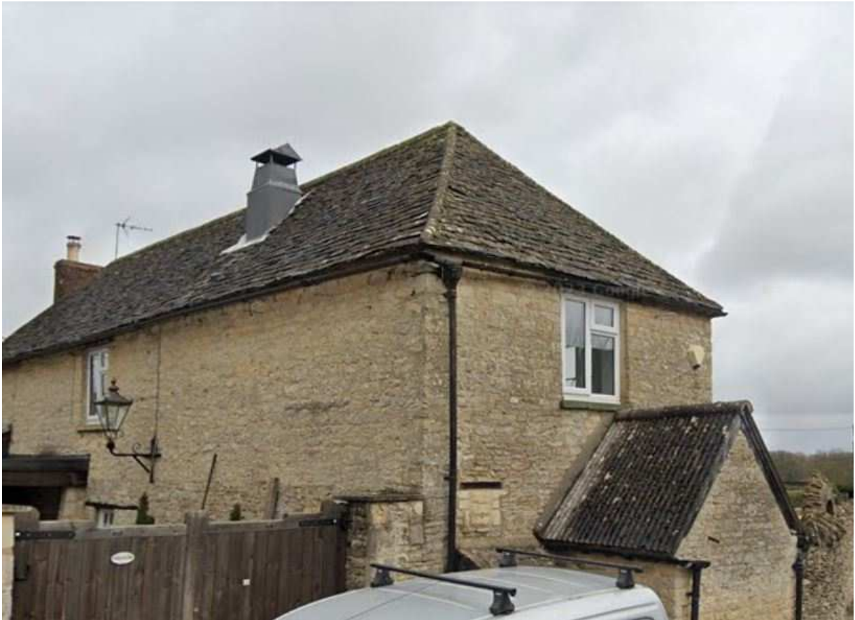
Fig 6. Kitchen extract chimney to be removed from East-facing roof slope
