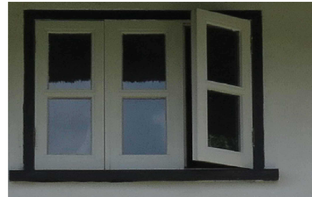
Images of the Existing Windows on North - East Elevation
