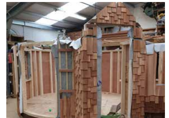
Use of prefabricated timber frame to minimise construction waste
