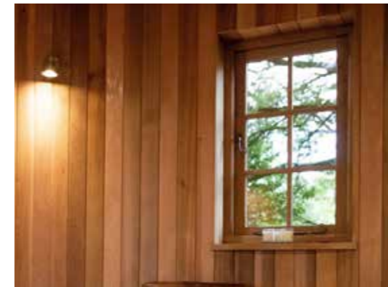
Double glazed 'plastic free' timber windows
