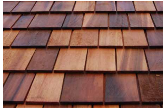
1. Cedar shingle roof
