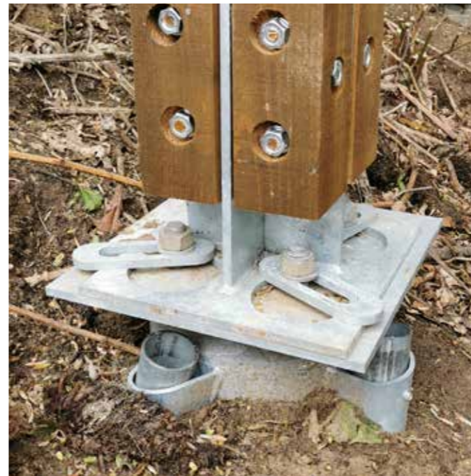
4. ROOT PILE CAP WITH POST ANCHOR
