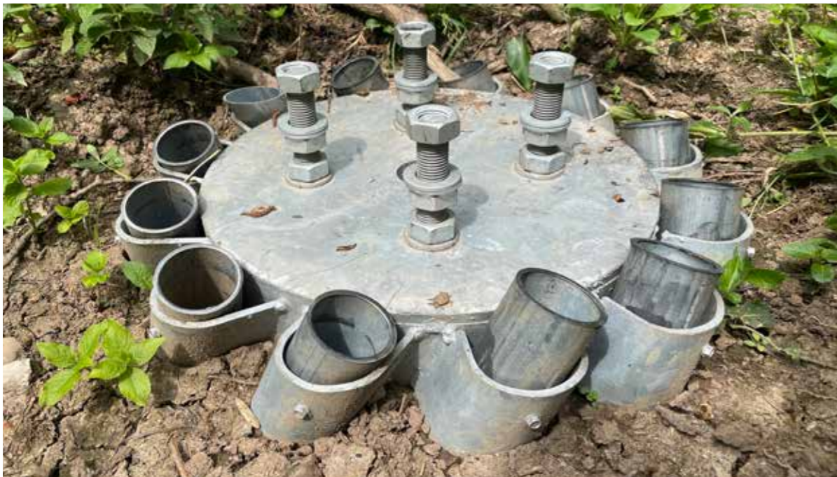
3. ROOT PILE CAP DETAIL
