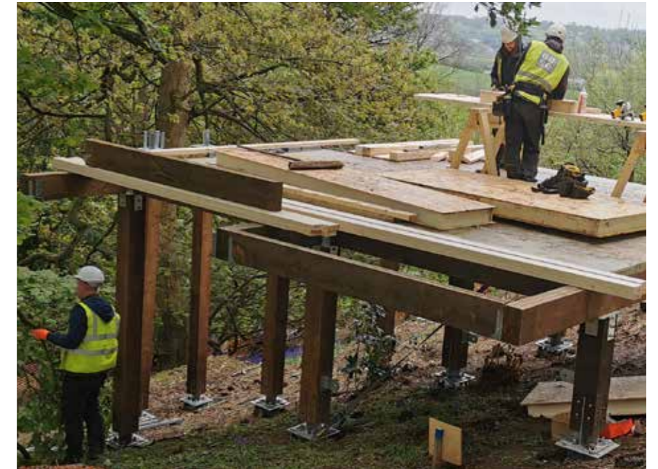
5. BUILDING FRAME ERECTED ON PILE CAPS
