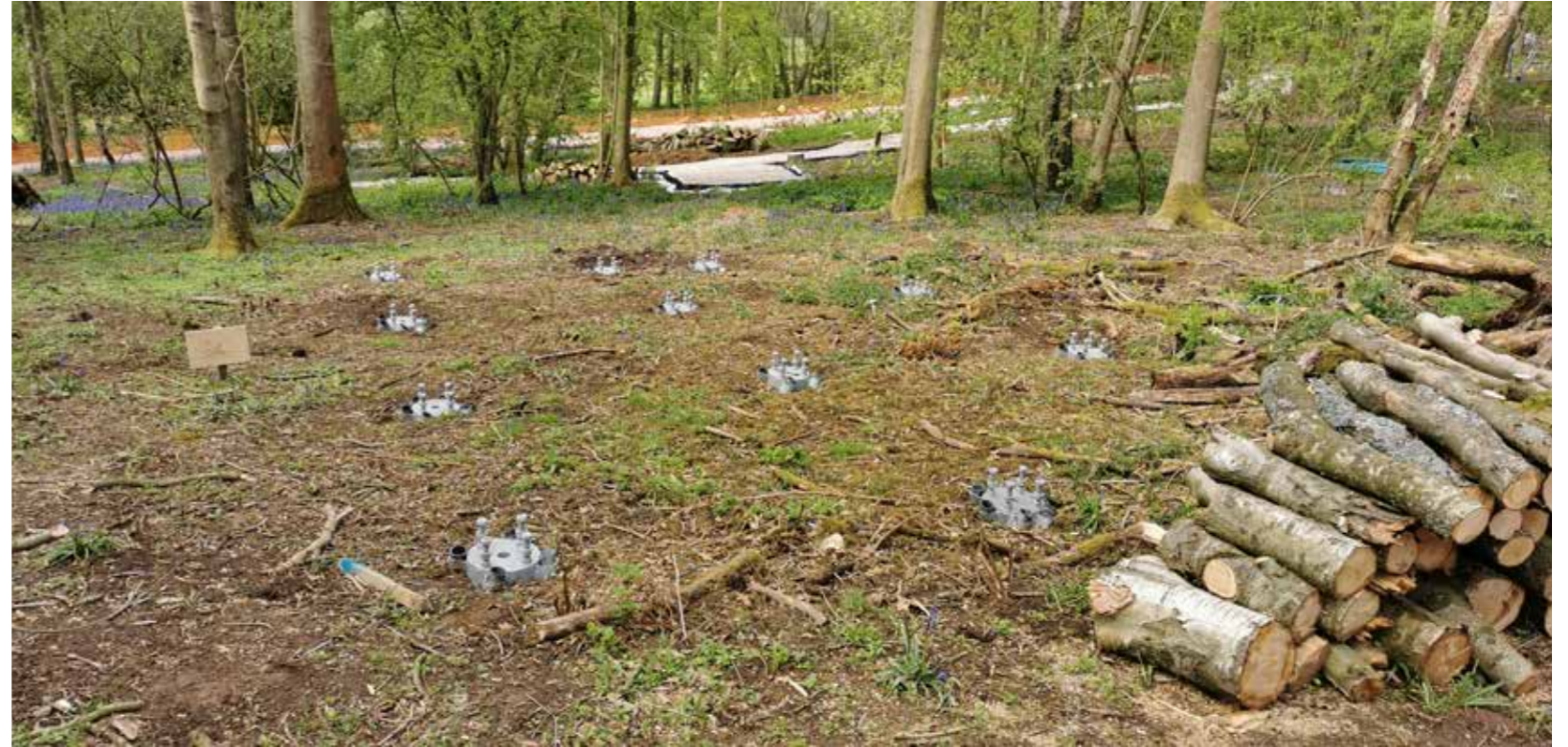
2. ROOT PILES INSTALLED
