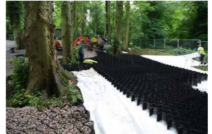
IMAGE A - CELLWEB GROUND PROTECTION
