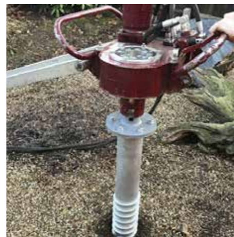
GROUND SCREW PILE
