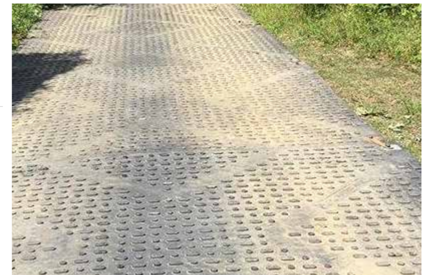
IMAGE B - TEMPORARY GROUND MATS
