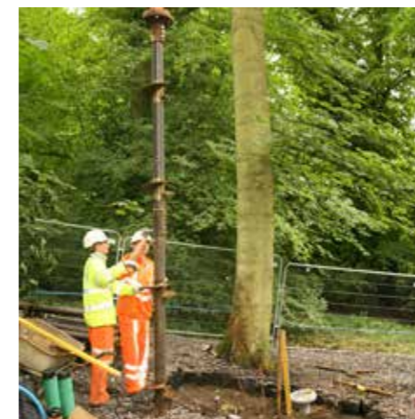
HELICAL SCREW PILE
