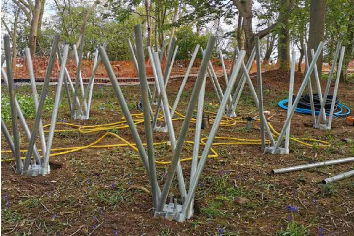
1. ROOT PILES SET OUT FOR INSTALLATION
