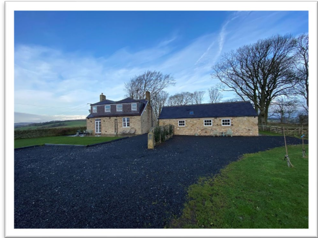
Figure 7 Laverick Cottage and the Bothy looking north
