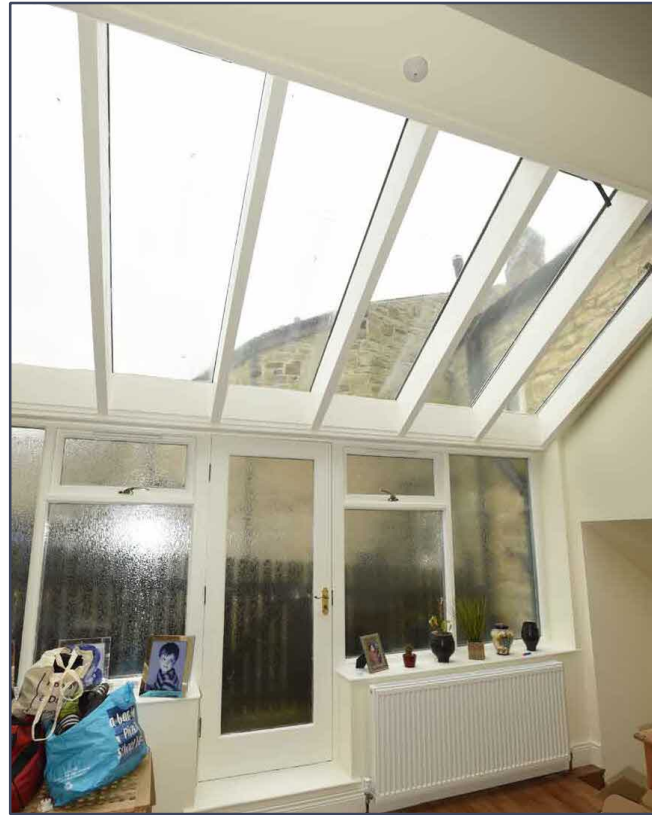
Existing East Elevation, Roof Glazing & External Door
