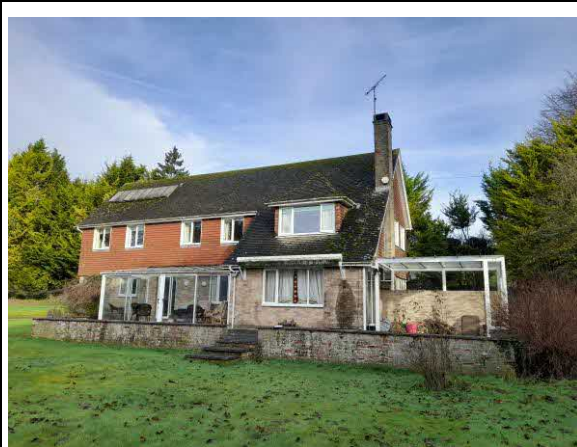
Photograph 1. General view of the southern elevation of the dwelling.
