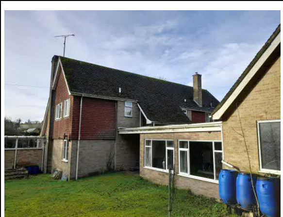
Photograph 2. Northern and eastern elevations of the dwelling, and eastern elevations of the extension adjoining to the garage.
