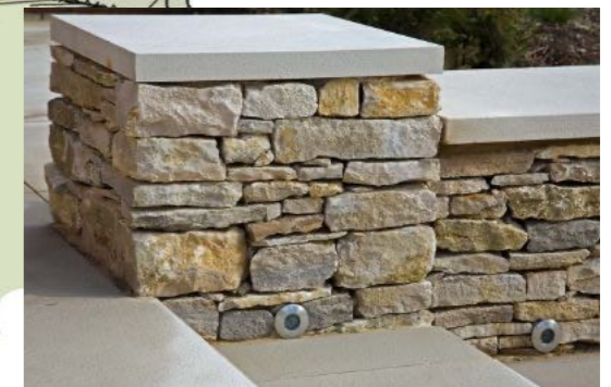
Limestone coping over low stone retaining walls
