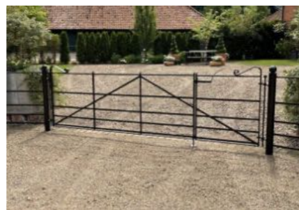
Estate gates and railings near house timber post and rail elsewhere
