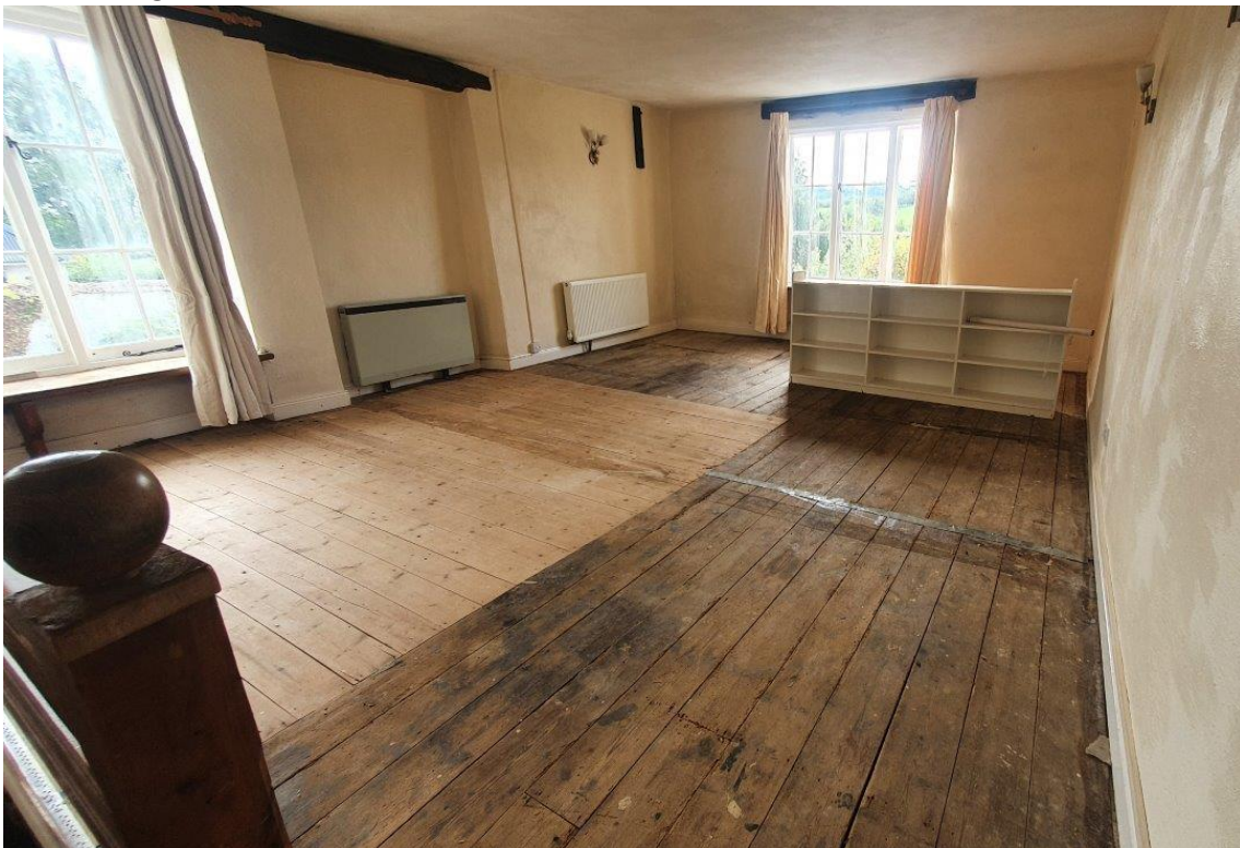
Existing large first floor room.
