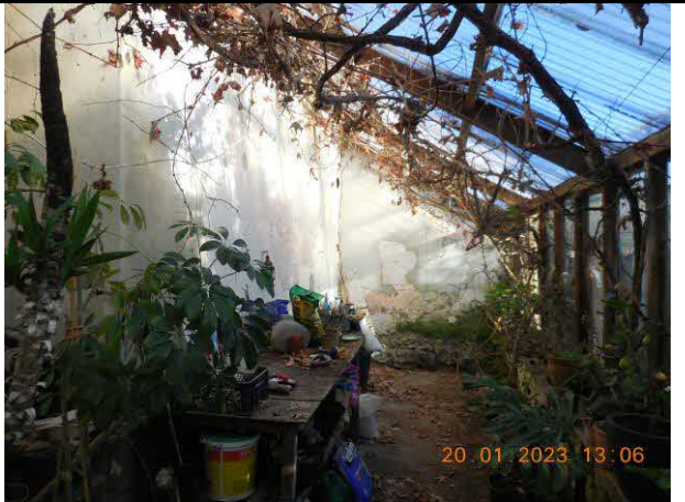
Plate 4. The interior of the conservatory on the southern elevation
