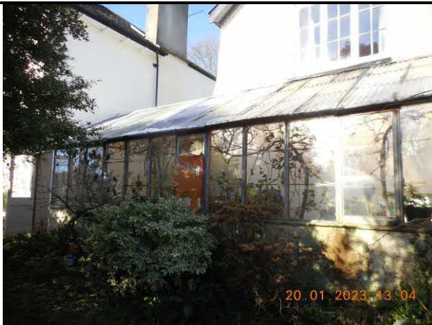
Plate 2. The southern elevation of the area surveyed looking west
