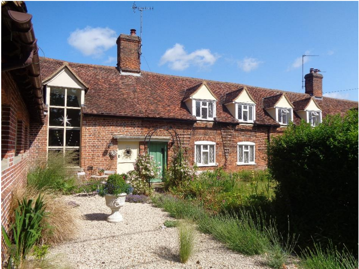
Street frontage of former school and almshouses
