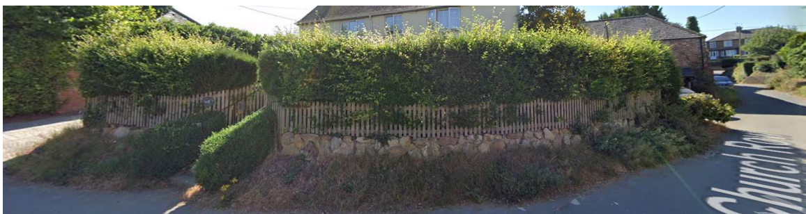
Boundary walling – Church Row
