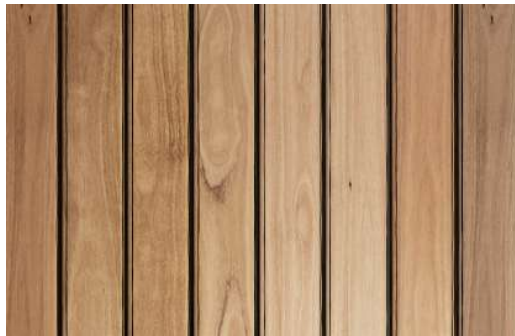
Vertical timber cladding
