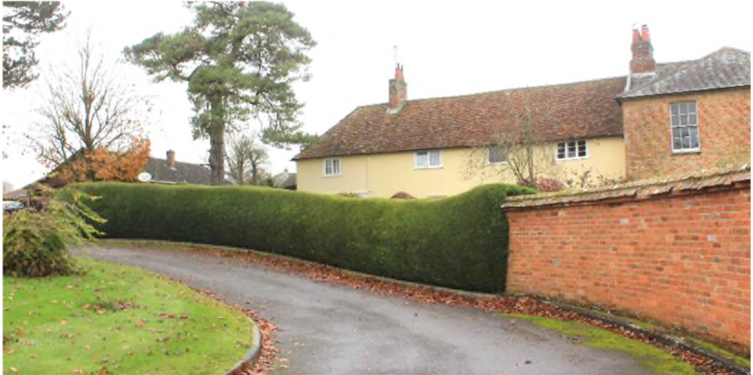
Figure 7 The view to the east gable of the main range and rear range of the Manor House is seen from the lower part of Church Close with Edelweiss beyond the left.
