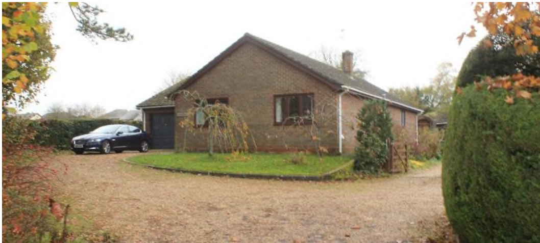
Figure 8 Edelweiss, east and north elevations.
