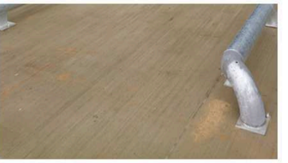
Insitu concrete yard
