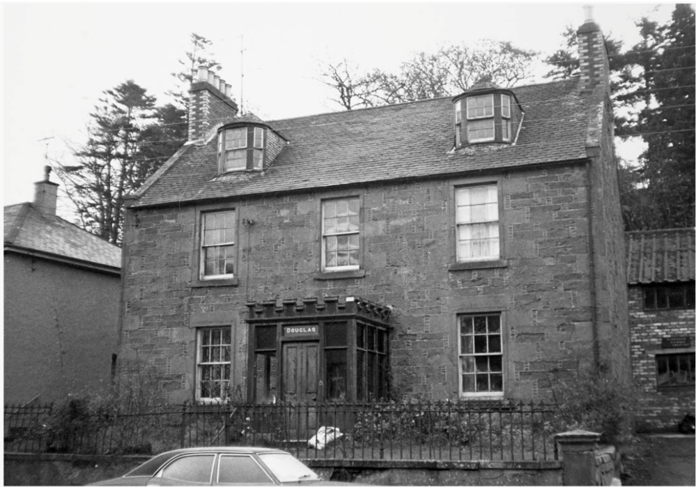
Δ Photograph from Canmore circa 1976 showing the original porch & railings
