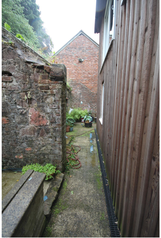
↑ View along rear of house looking South
