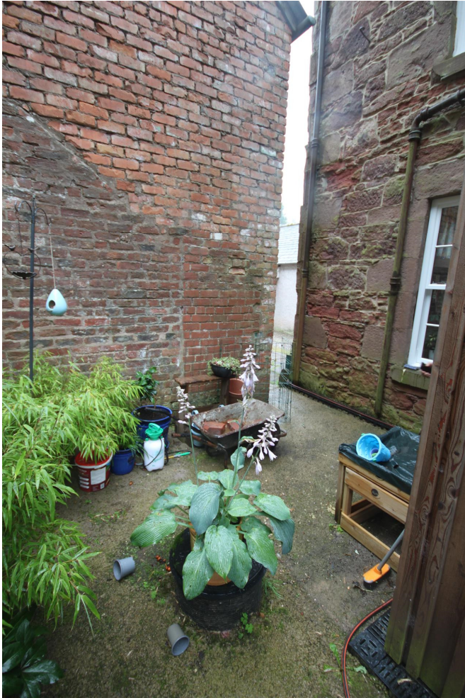
↑ View of rear of house & garage gable
