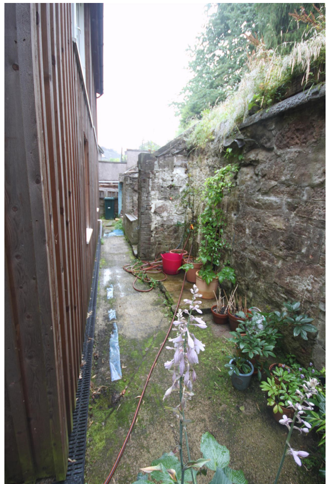
↑ View along rear of house looking North
