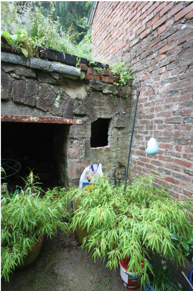
↑ View of wall to rear of house & garage gable
