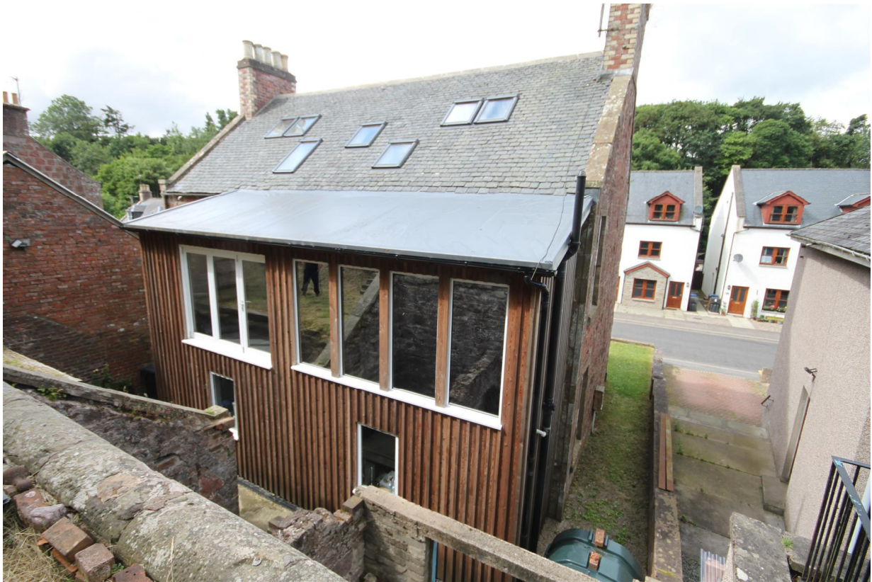
↑ View of two storey rear extension from garden at high level
