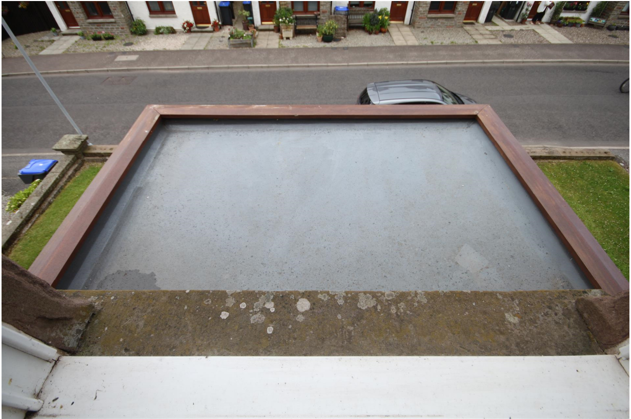
↑ View of porch roof from first floor bedroom window
