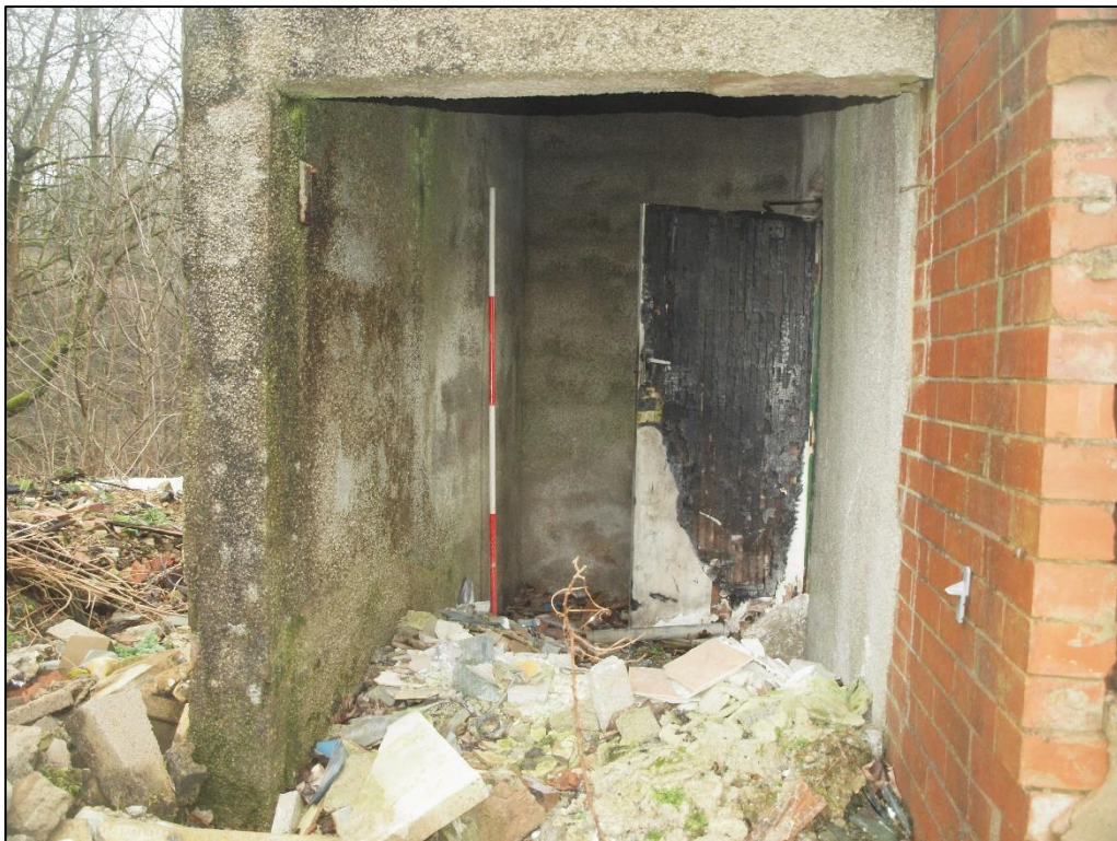
Plate 28: As above looking west
