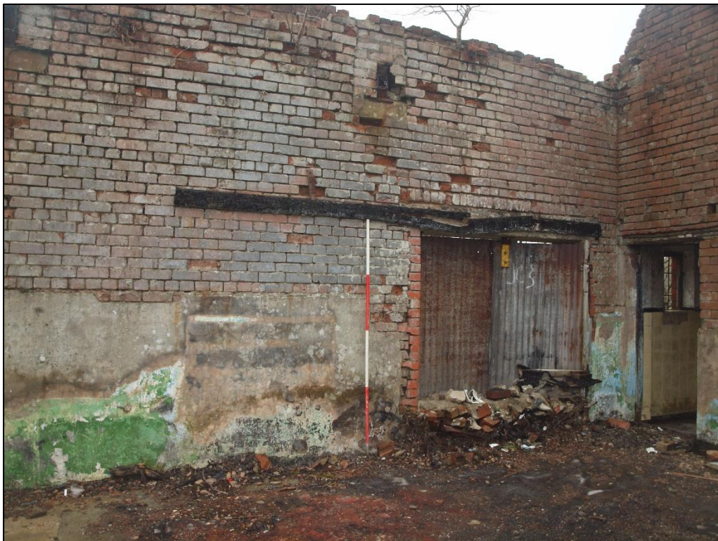
Plate 34: North end of west wall showing loading doorway with burnt lintel
