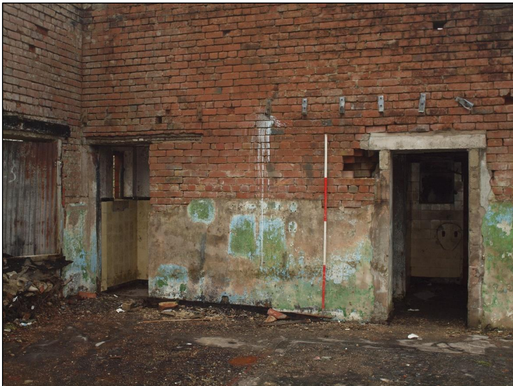
Plate 36: Detail of doorways to west side
