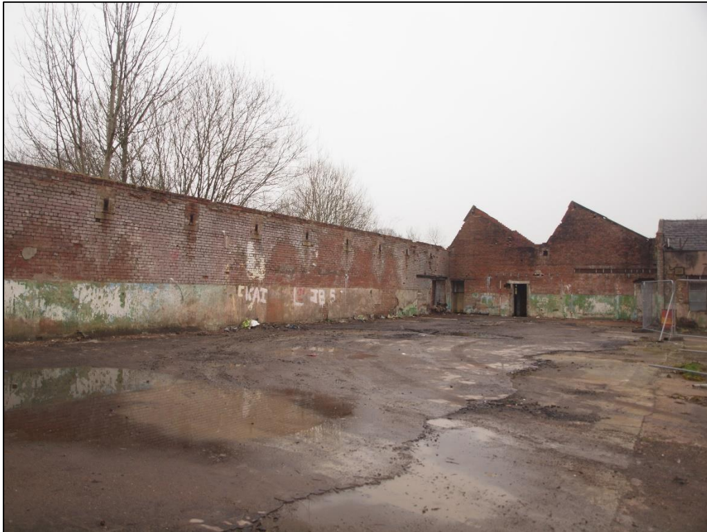
Plate 33: North internal gable and west wall
