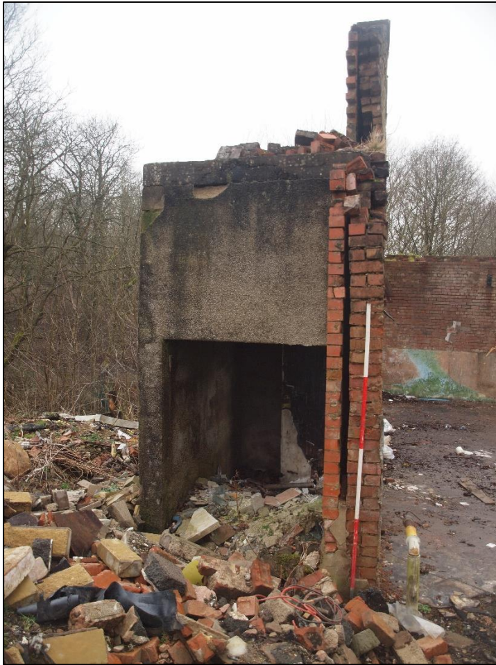
Plate 19: Remaining east elevation of southern extension
