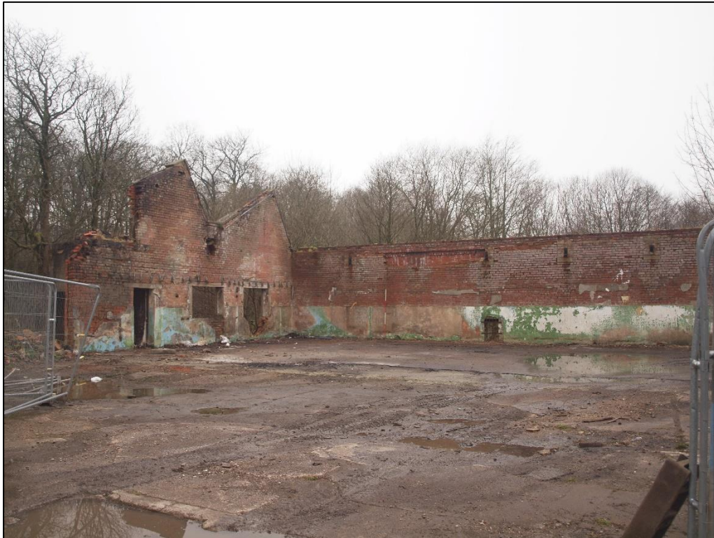
Plate 1: General shot of Building from the east
