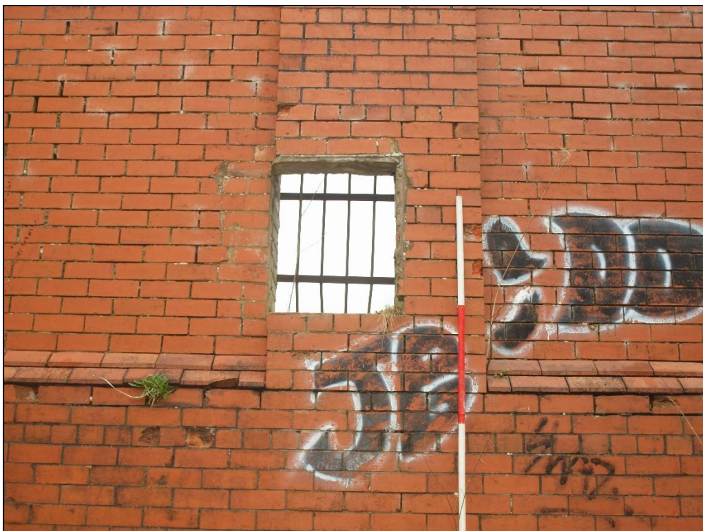
Plate 10: Inserted opening
