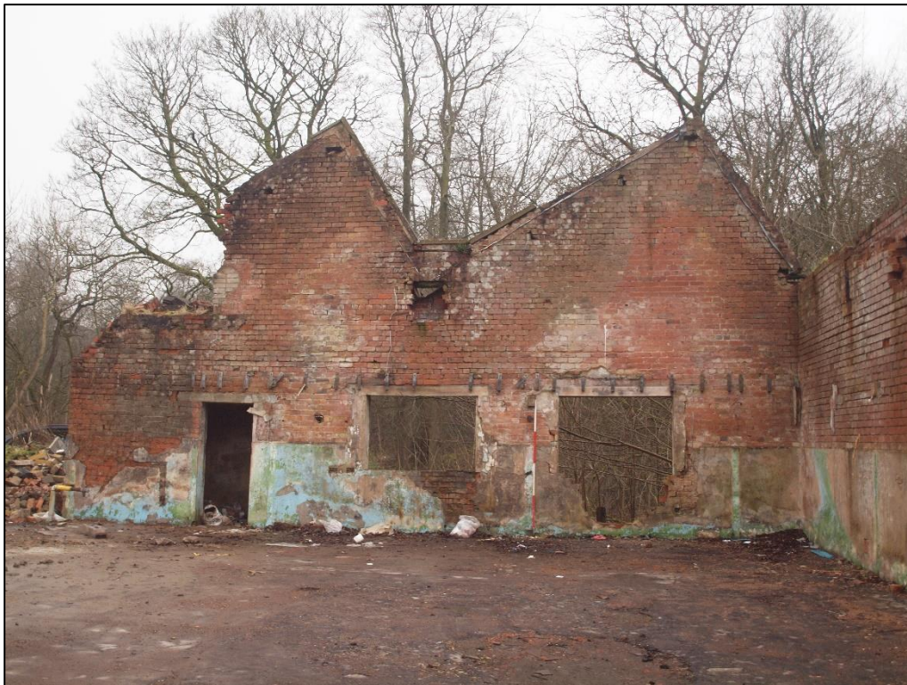
Plate 20: Internal southern gable
