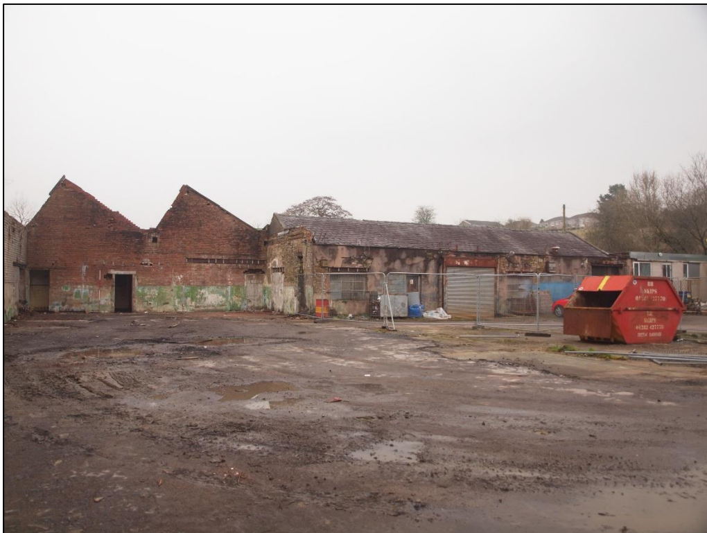
Plate 2: General shot of the site looking north
