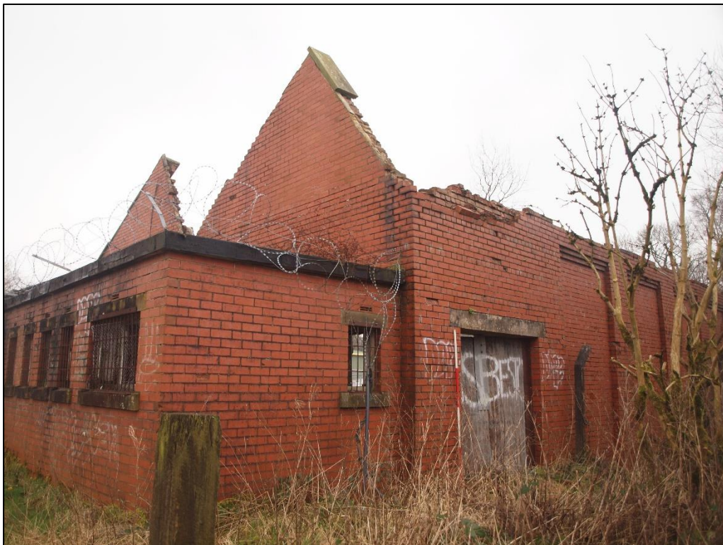
Plate 12: North end of west elevation
