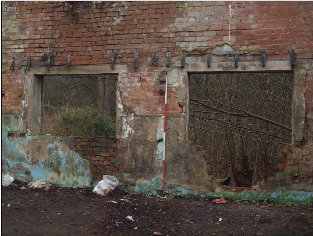
Plate 21: Detail of large windows
