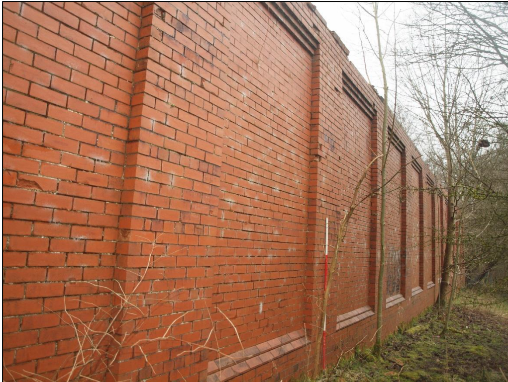
Plate 11: North end of west elevation looking south
