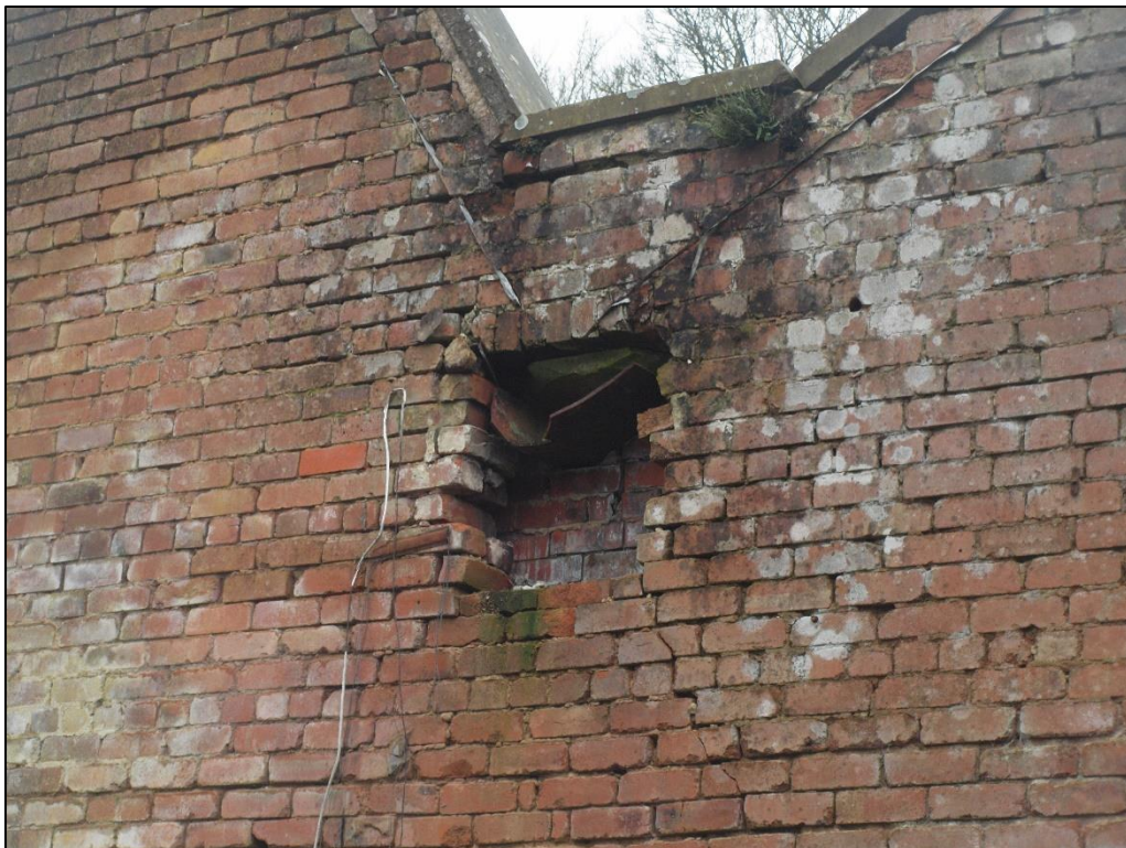
Plate 22: Opening showing where guttering was located
