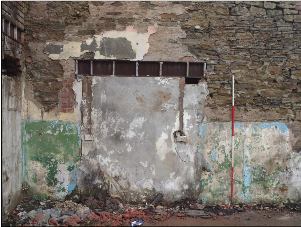
Plate 45: Detail of blocked doorway shown above
