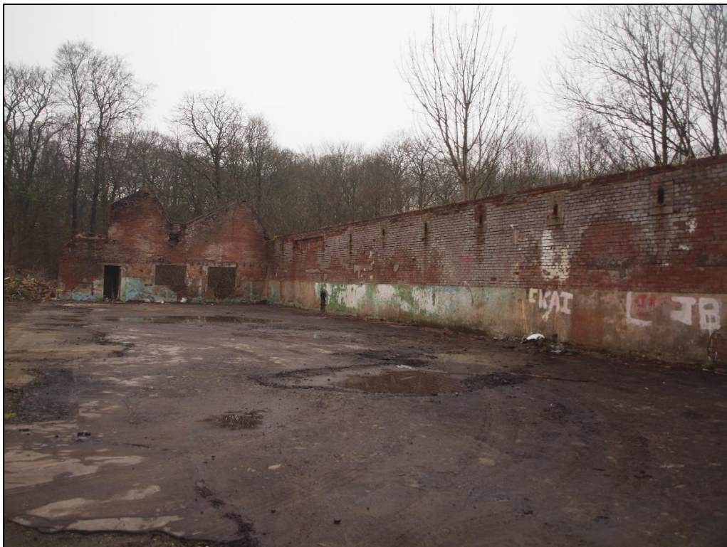
Plate 30: Southern internal gable and internal west wall
