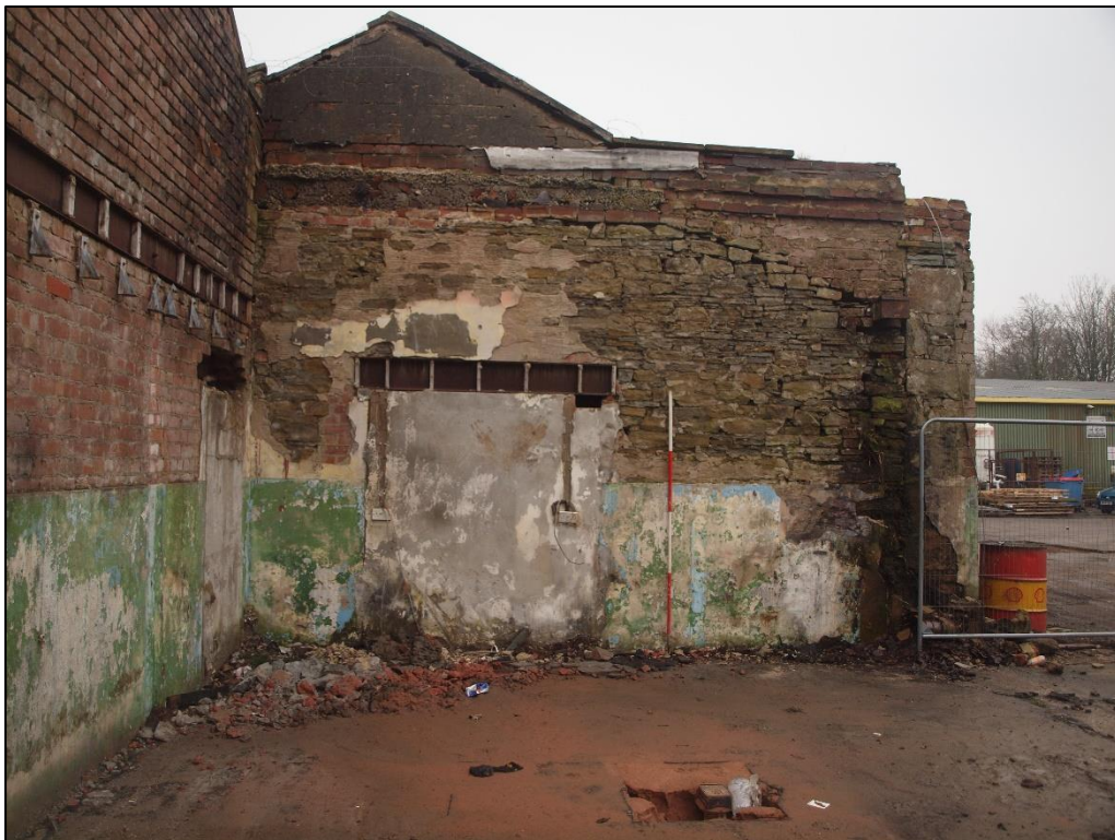
Plate 44: Remaining internal east elevation showing stone construction of adjoining building
