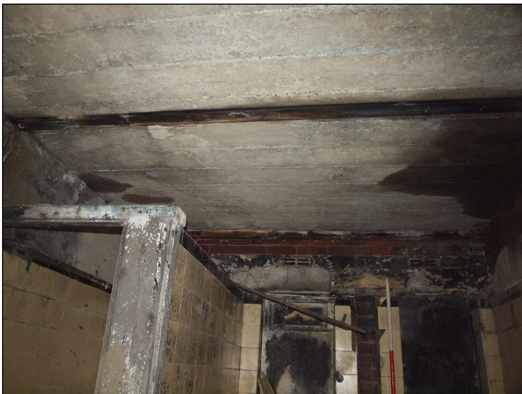
Plate 40: Concrete ceiling detail
