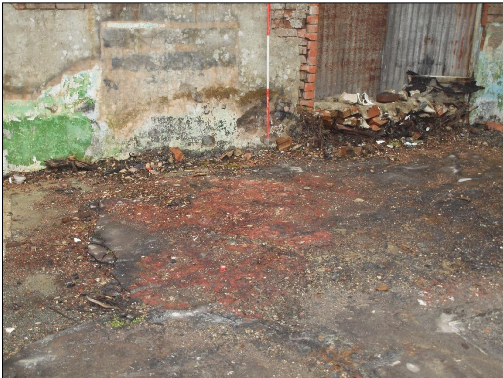
Plate 38: Patch of brick flooring to northwest corner
