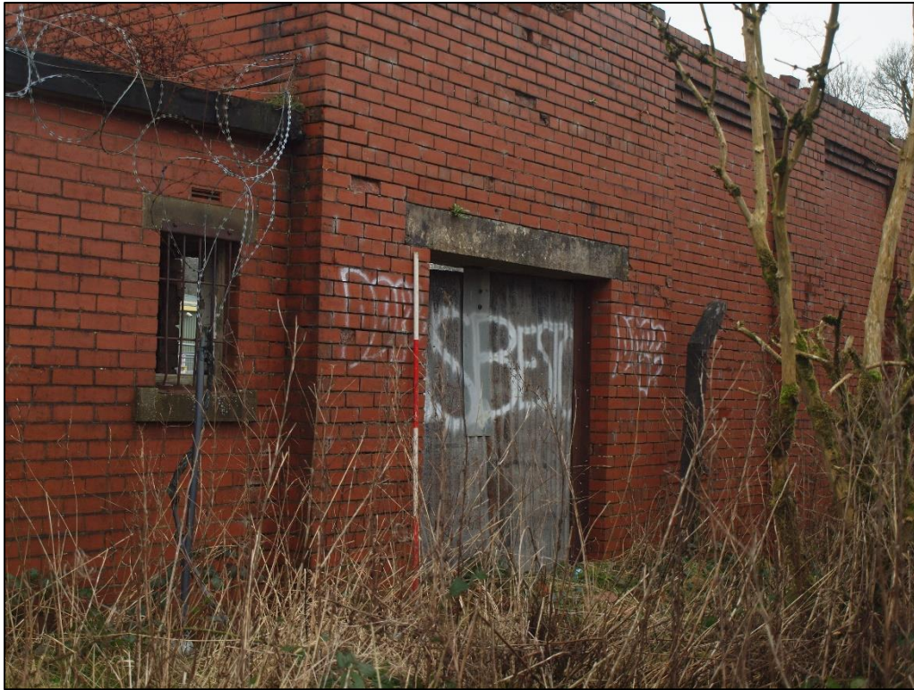
Plate 13: Detail of loading door and window to toilet block
