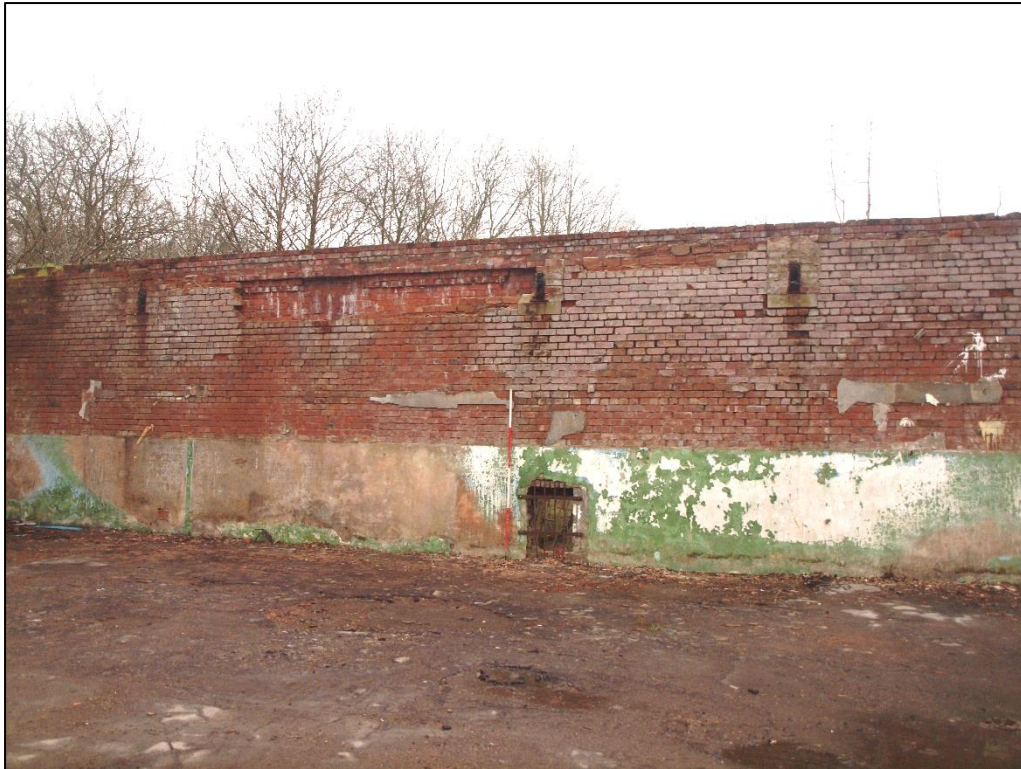
Plate 31: South end of west wall showing opening and beam slots above
