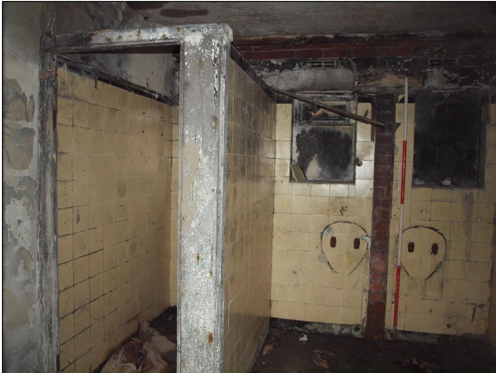
Plate 39: Interior of toilet block, east side
