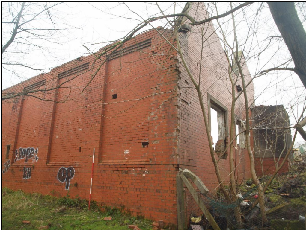
Plate 8: South end of west elevation
